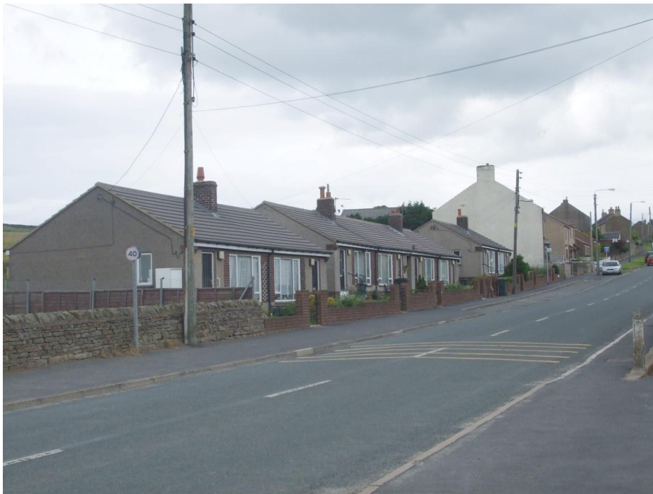
Figure 15 Terraced Housing Association Bungalows in a Teesdale Village
