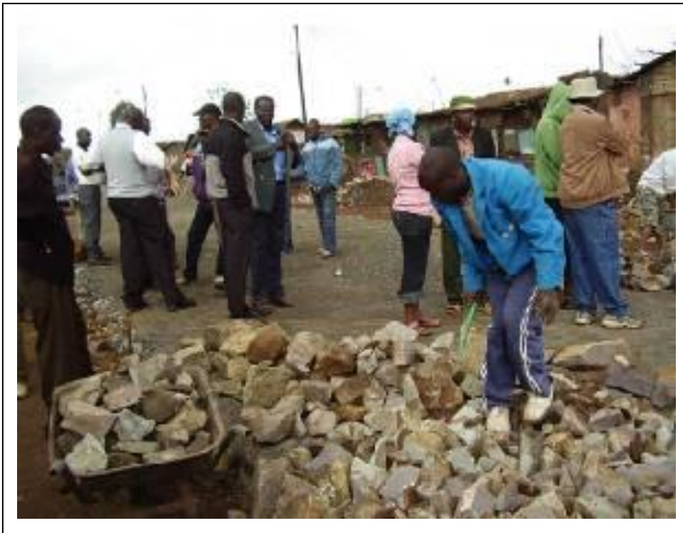
Figure 7-18 Korogocho Youth Engaged in Road Construction
