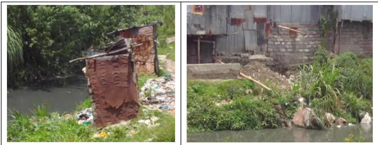
Figure 7-21 Toilet Structures Located Adjacent to the Ngong River Note the pipes emptying into the river
