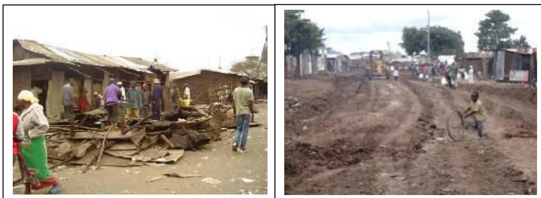
Figure 7-11 Structure Removal in Korogocho to Pave way for Road Construction
