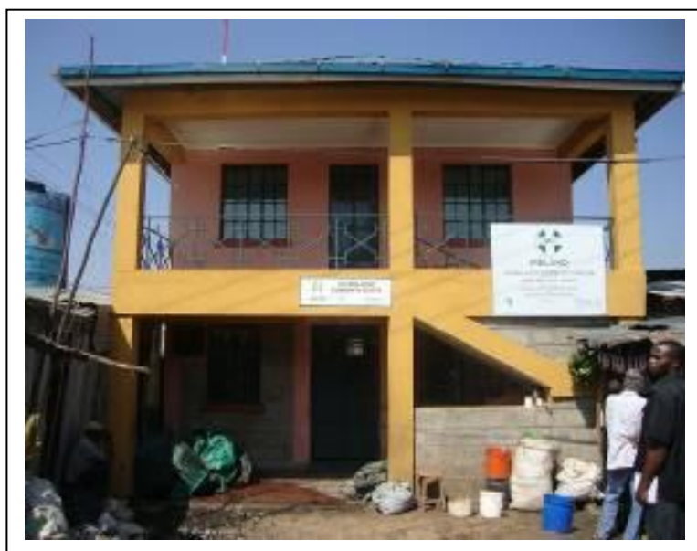
Figure 5-9 Sanitation block constructed in Mukuru
