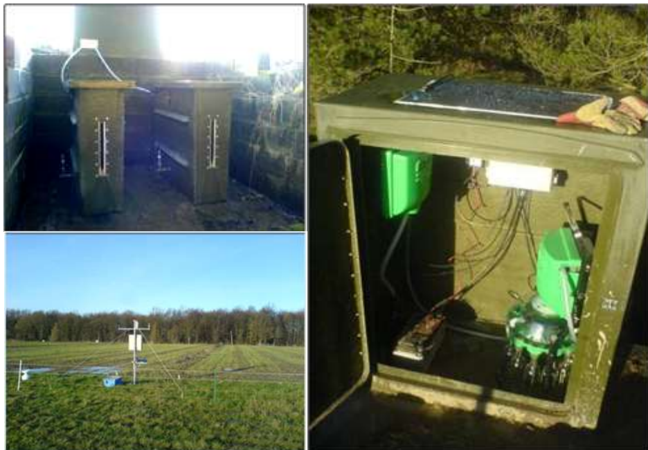
Photo 3.2: Clockwise from top left: flow monitoring box weirs; water samplers; automated weather station with plots in background.
