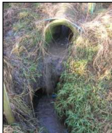
Photo 2.13: Track runoff (top) entering the experimental ditch.
