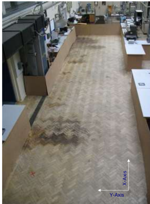
Figure 7.1: Robotics and Automation Research Labortary, Newcastle University (including hard-board panels)
