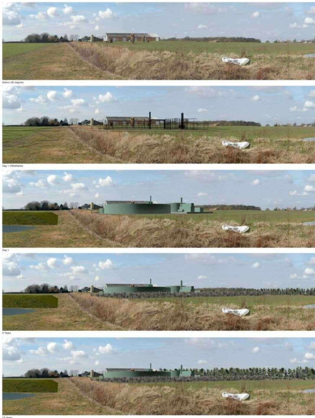
Figure 6.2 Typical Photomontage Productions – Existing, Wireframe, Day 1, Year 5 and Year 15 (Courtesy of AWP Ltd, 2010)
