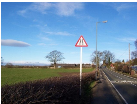
Figure 4.17 Existing Site Photograph (Windlestone Hall School Site)
