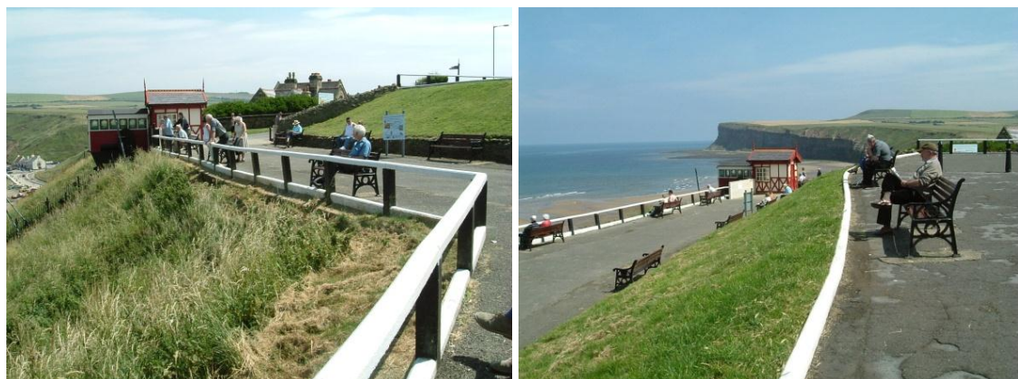
Figure 4.14 Site Photos - Exiting Cliff Lift (Before construction)
