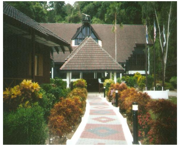
RMPc administration and information building
