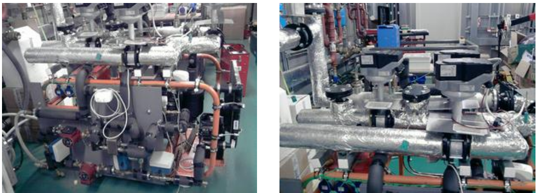
Fig. 3.12 Waste heat recovery system
