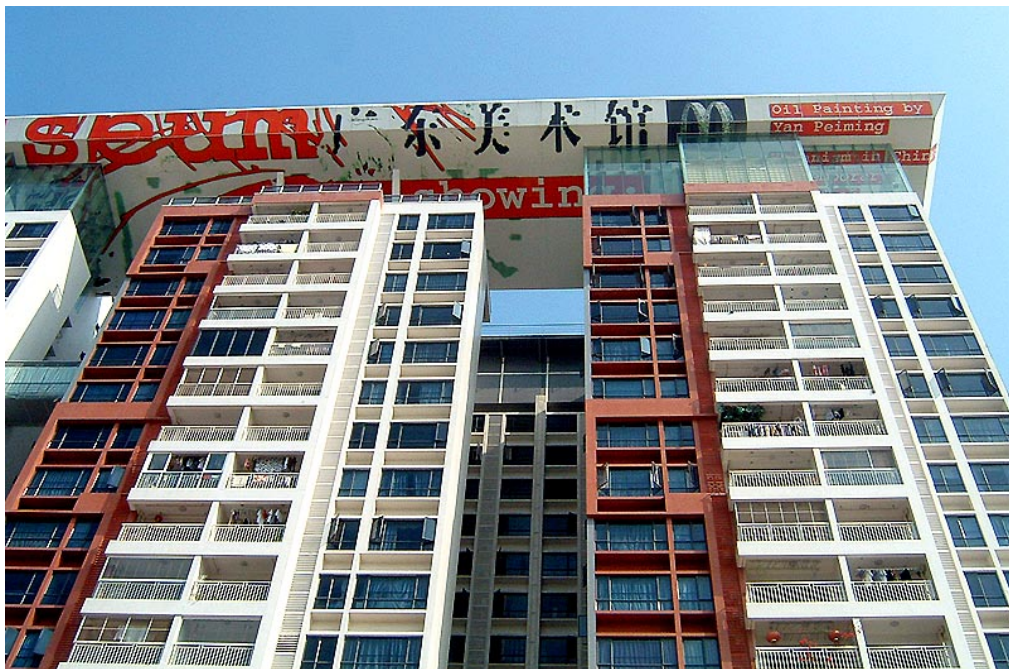
[Figure 40] The new site of the Times Museum, GDMOA Photo: Y.J. Chen
