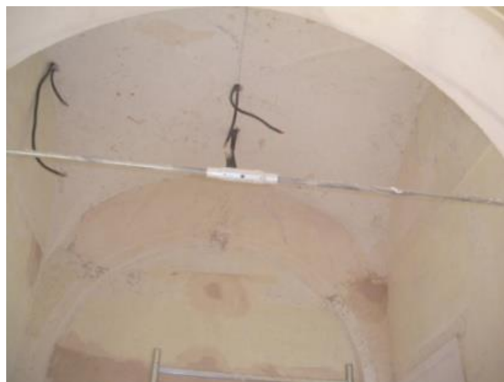
Figure 6.14: Pre-stressed metals to prevent horizontal force in the Islamic museum’s arches (the author, 2010)
