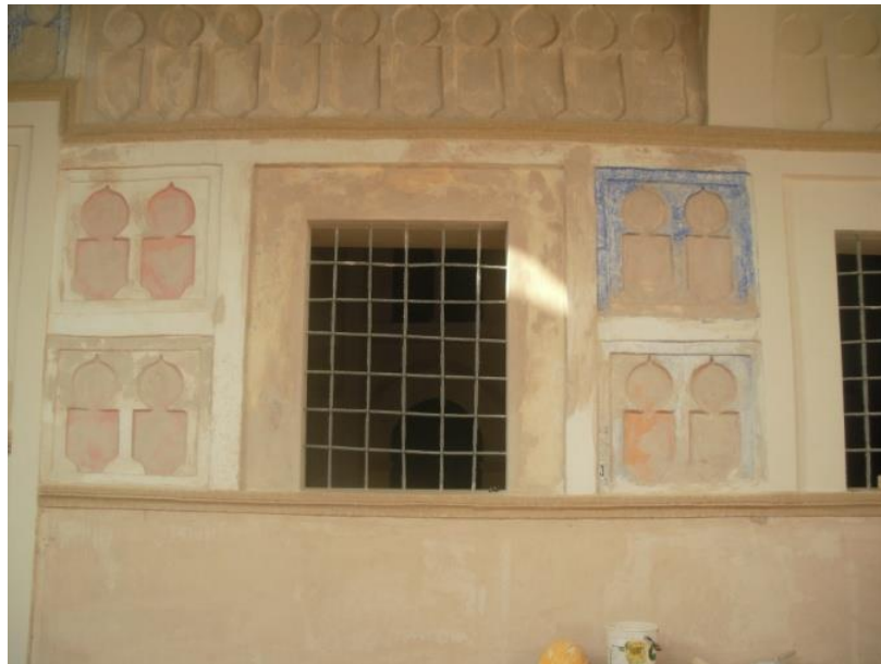
Figure 6.5: removing layers of old paint in the Islamic museum, Tripoli (the author, 2010)
