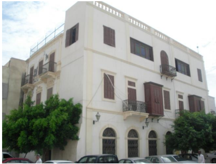
Figure 5.4: The former Bank of Rome in the old city of Tripoli (the author, 2010)
