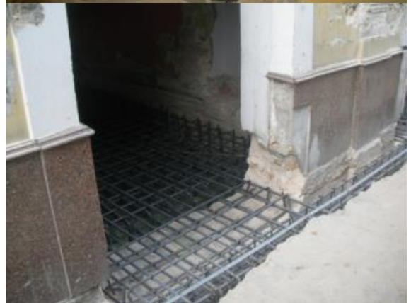
Reinforced concrete was used to consolidate the foundations
