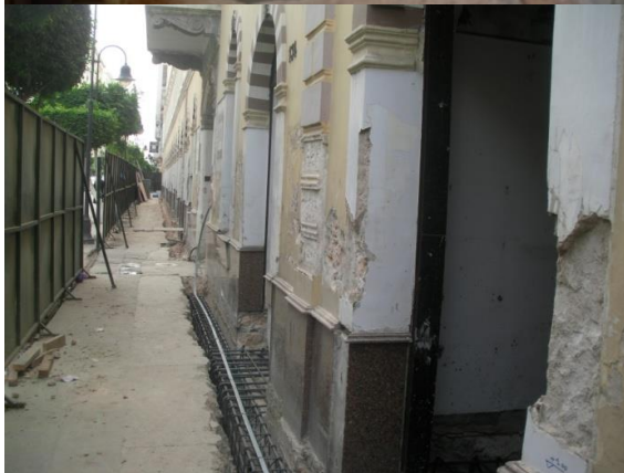
Reinforced concrete was used to consolidate the foundations
