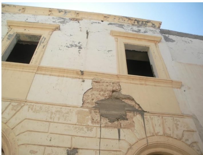
Figure 6.13: Concrete keys used to repair wall cracks, Tripoli (the author, 2010)
