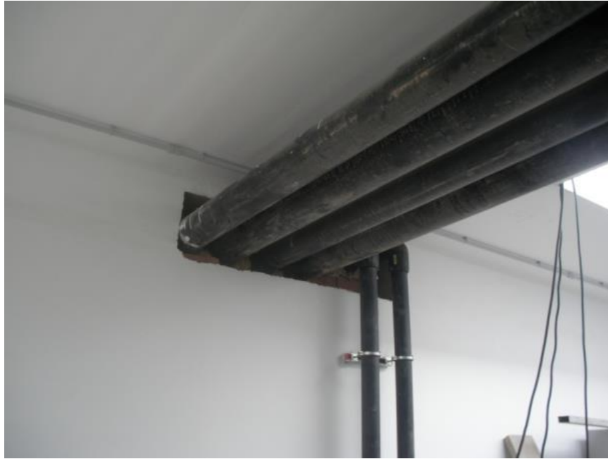
Figure 6.7: underground services in the Islamic museum in Tripoli (the author, 2010)
