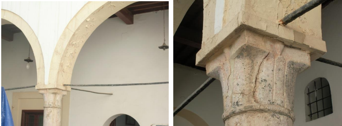
Figure 6.15: The wrong type of metal was used in the former British consulate in Tripoli (the author, 2010)
