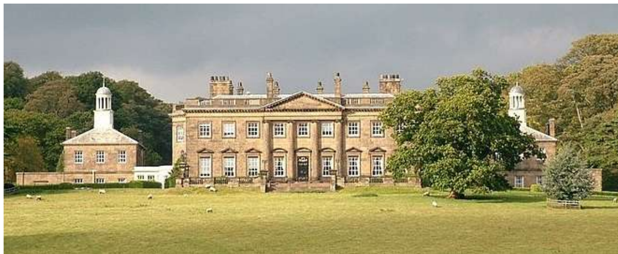
Figure 6.3: Denton Hall, North Yorkshire, by John Carr, 1772-78.
