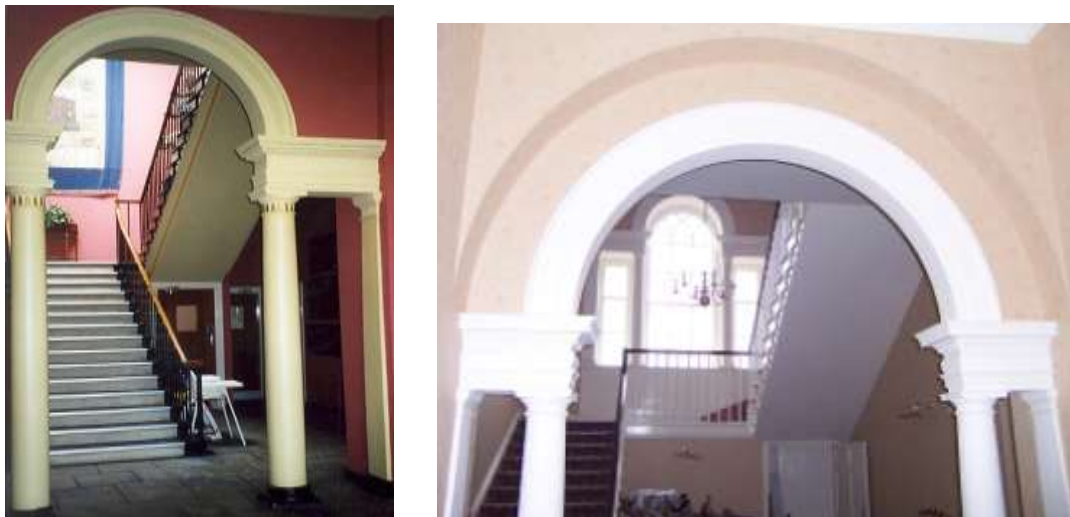
Figure 7.20: Comparison of Serliana staircase screens at Backworth Hall (1778) and Newton Hall, Newton-by-the-Sea (attributed to William Newton).
