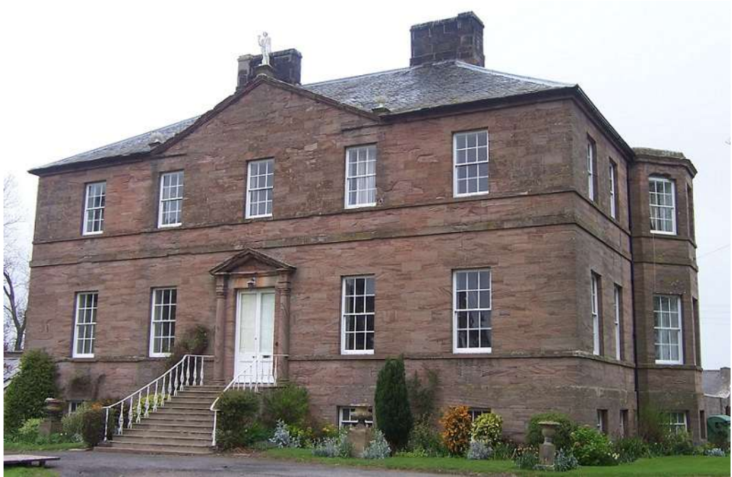
Figure 7.33: Newton Hall, Newton-by-the-Sea (Northumberland). Villa with services in basement (note windows at ground level), family rooms on piano nobile with canted bay window looking towards the coast, upper floor for family bedrooms and servants' accommodation in attics.
