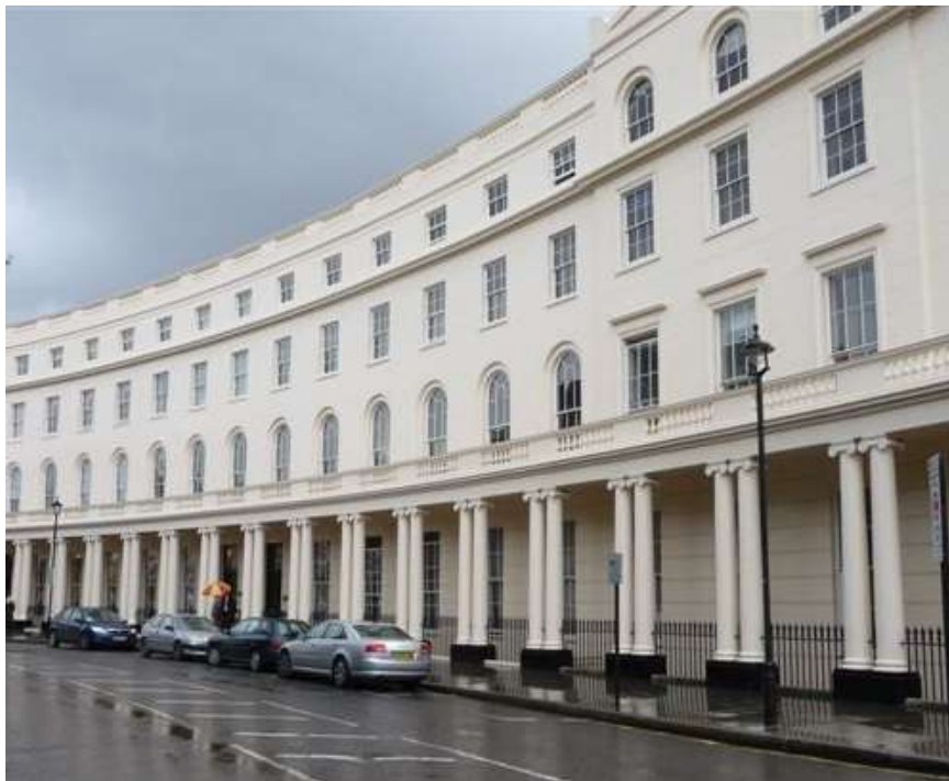
Figure 7.25: Park Crescent, London, by John Nash, 1806, showing stuccoed brick scored to imitate stone construction.
