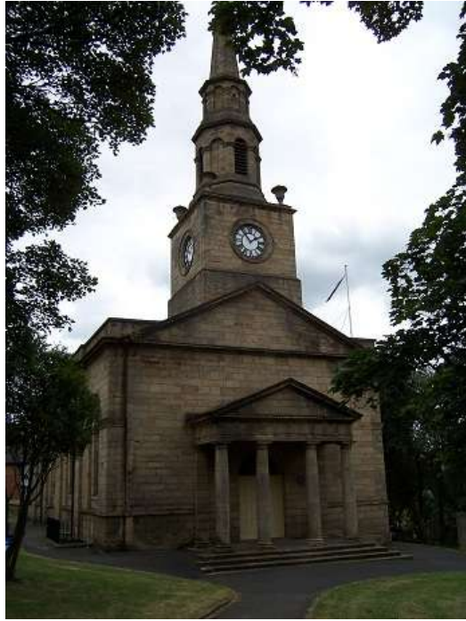
Figure 7.11: Chapel of St. Ann, Newcastle by William Newton, 1764-1767. View from the west.
