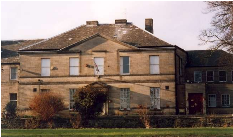
Figure 8.9: Benton House (Northumberland), home of Thomas Charles Bigge, architect unknown
