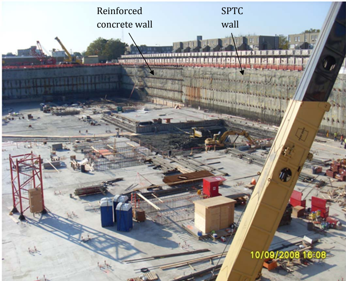
Figure 6.4: SPTC wall and conventional diaphragm wall
