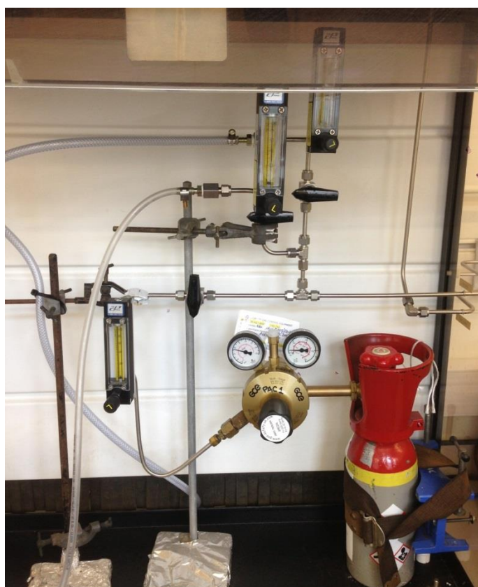
Figure 2.12. (a) Photograph of the FTIR spectrometer and pipelines used to control the flow rate and relative humidity of N_2 entering the environmental chamber. (b) Enlarged photograph of the gas pipelines.
