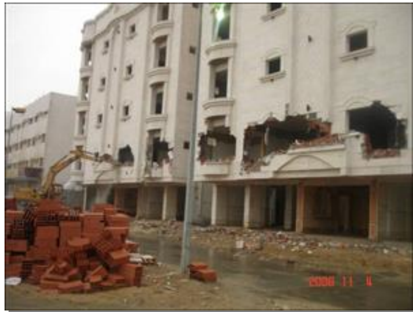
Figure 8.13: Removing the non-compliant part
