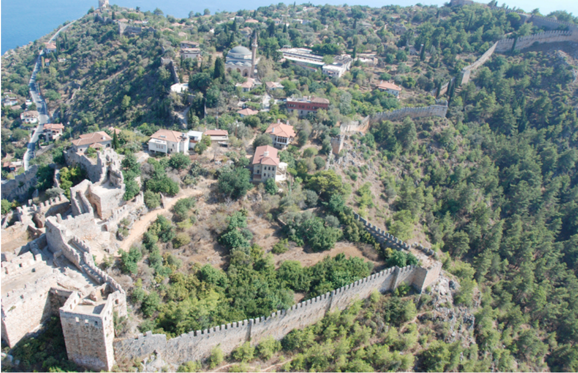
Figure 5.44: Alanya Castle. A partial view of Hisariçi featuring Süleymaniye Mosque (centre), Bedesten and Akşebe (Source: Alanya Municipality 2010)
