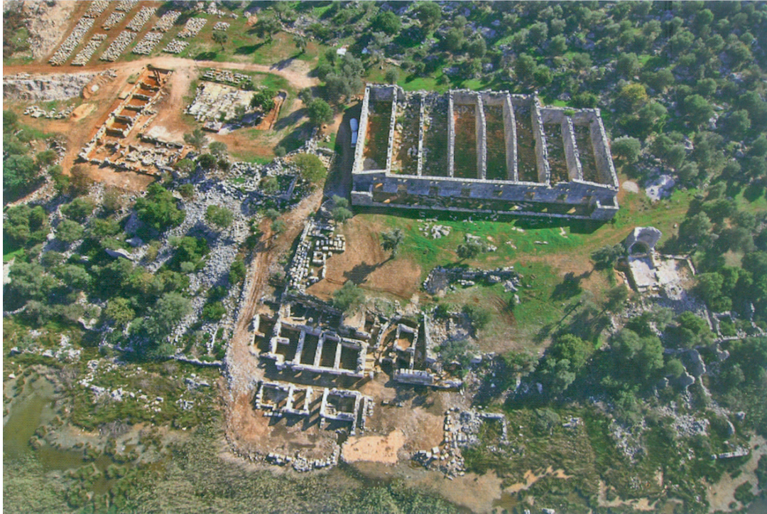
Figure 5.4: Andriake. The group of buildings featuring the Plakoma (top left) and the Granarium on its right hand side (Source: Çevik and Bulut 2010)
