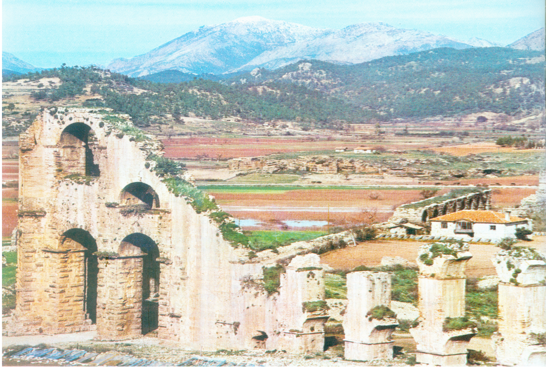
Figure 5.30: Aspendos. The Aqueducts (Source: Alpözen 1977)
