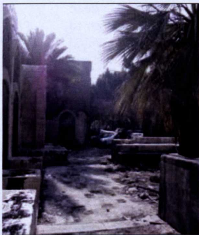
Fig 6.17 The deterioration in Abu EL-Dahab street
