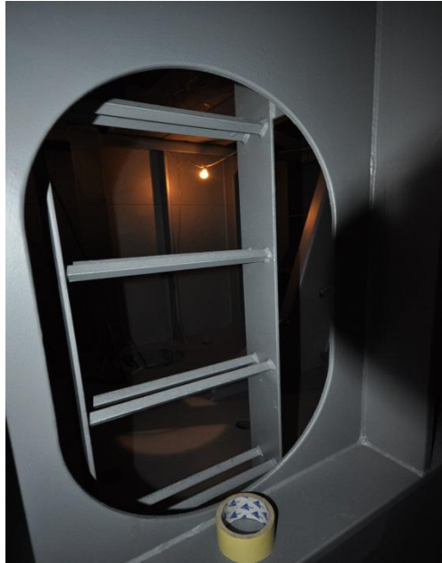
Figure 5-20 Ladders covering manhole
