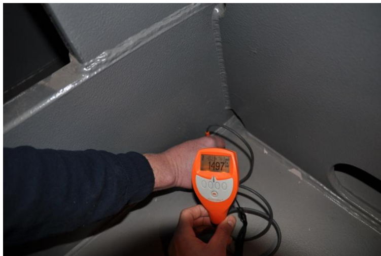
Figure 5-19 Example of Excessive Paint Thickness
