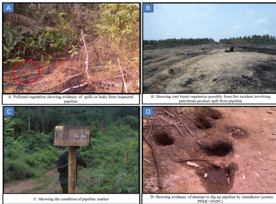
Figure 4-18. Condition of sample pipeline ROW
