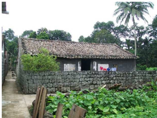
Figure 6.7 Traditional Hainanese house in Baili Baicun
