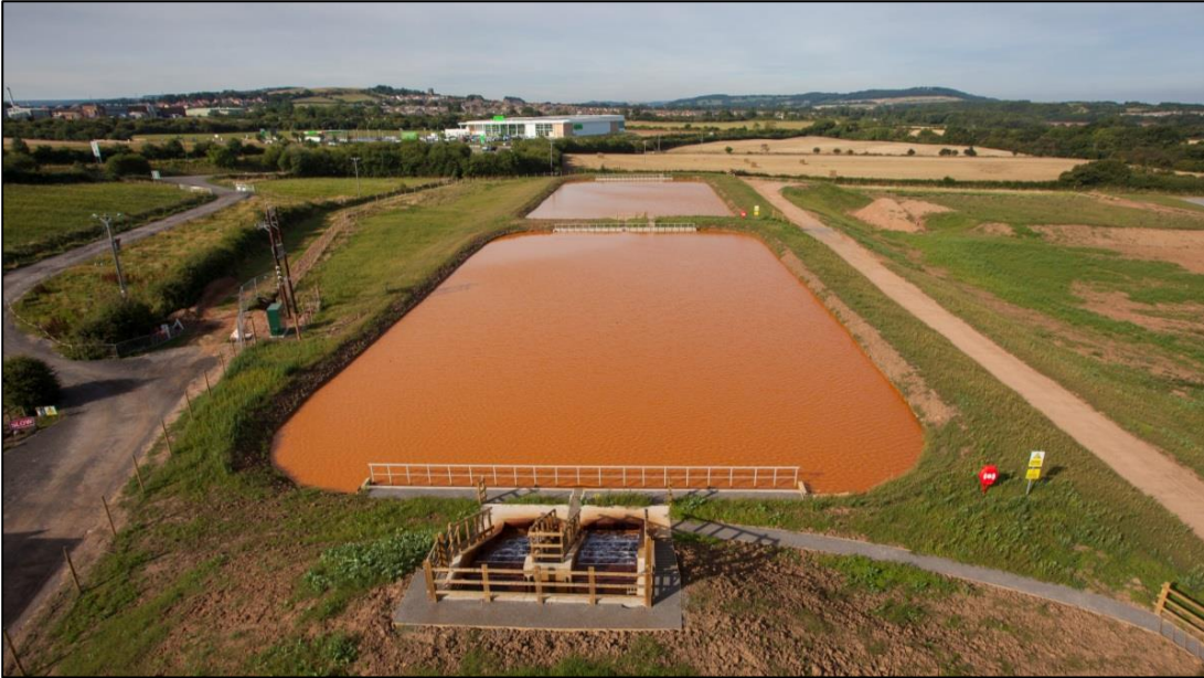
Figure 2.11 Saltburn passive treatment system tackling ferruginous mine water from ironstone workings (photograph courtesy of The Coal Authority)
