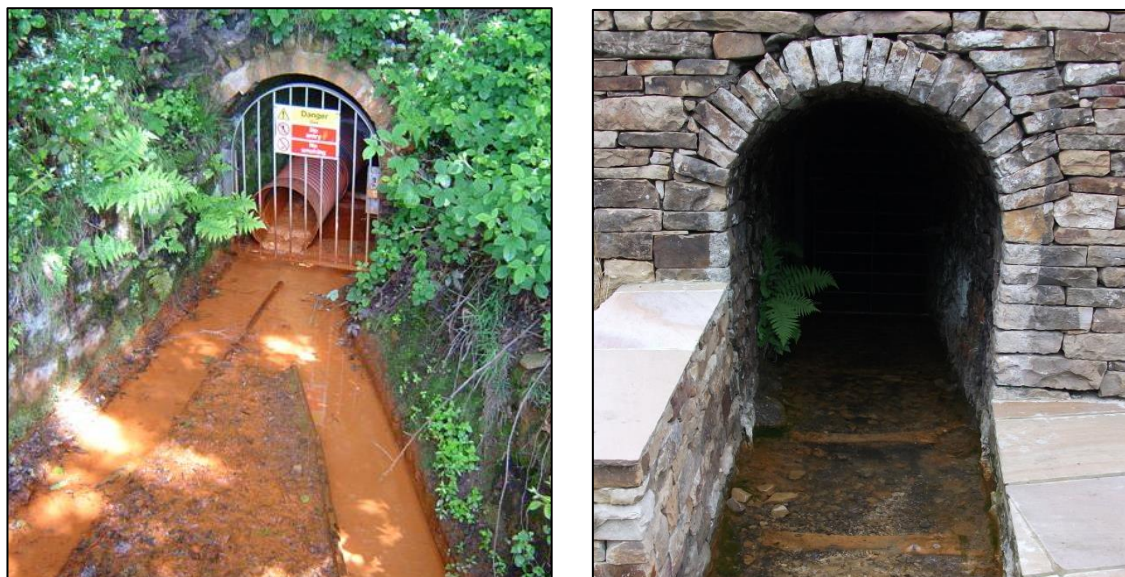
Figure 1.1 Ferruginous discharge at Handbank Colliery, Yorkshire, UK (left); and a metalliferous mine discharge with low iron concentrations, Nentsberry Hags Pb-Zn Mine, Cumbria, UK (right) (photographs courtesy of The Coal Authority).
