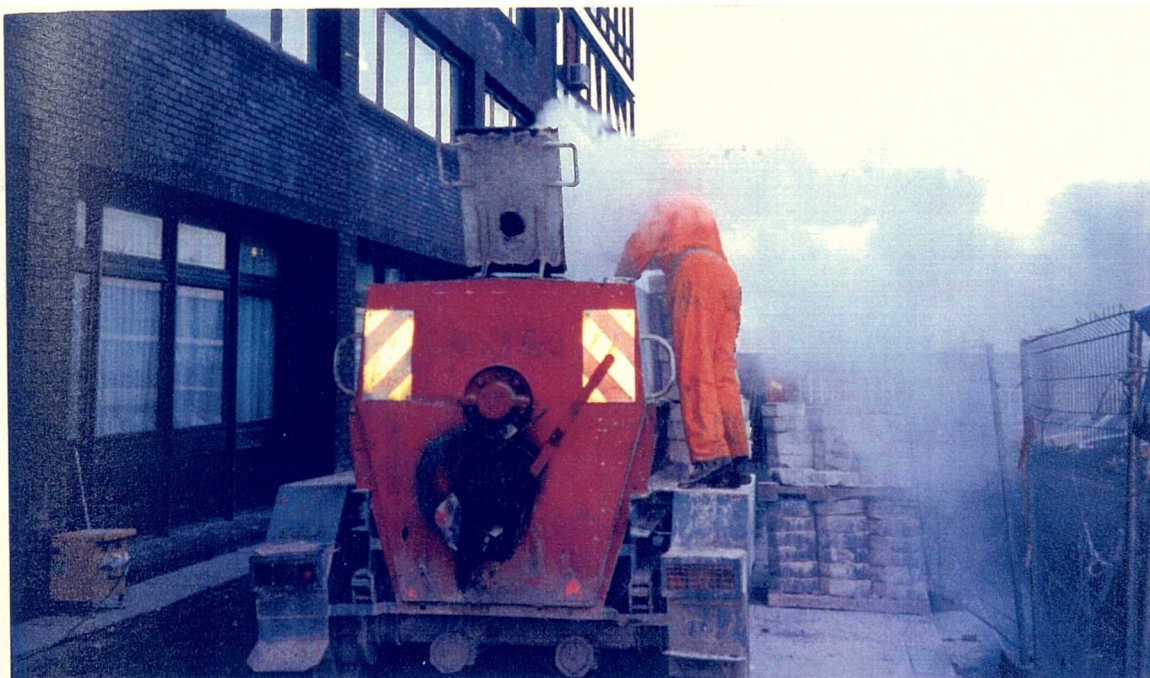
Figure : 11.2 b The Kettleman/mixer operator Feeding the Boiler With Mastic Asphalt Blocks
