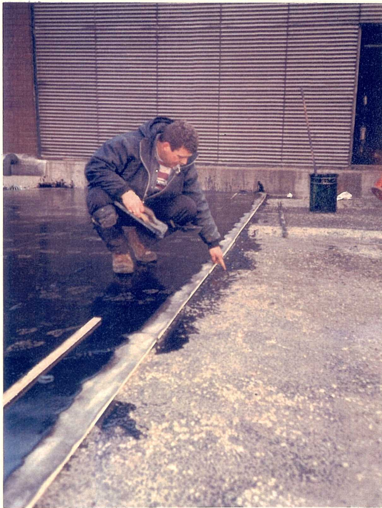
Figure : 11.2 a One of the Troweller Pointing at the Thin of Bitumen Film and the Glass-Fibre Mats Applied on Day One of Survey D
