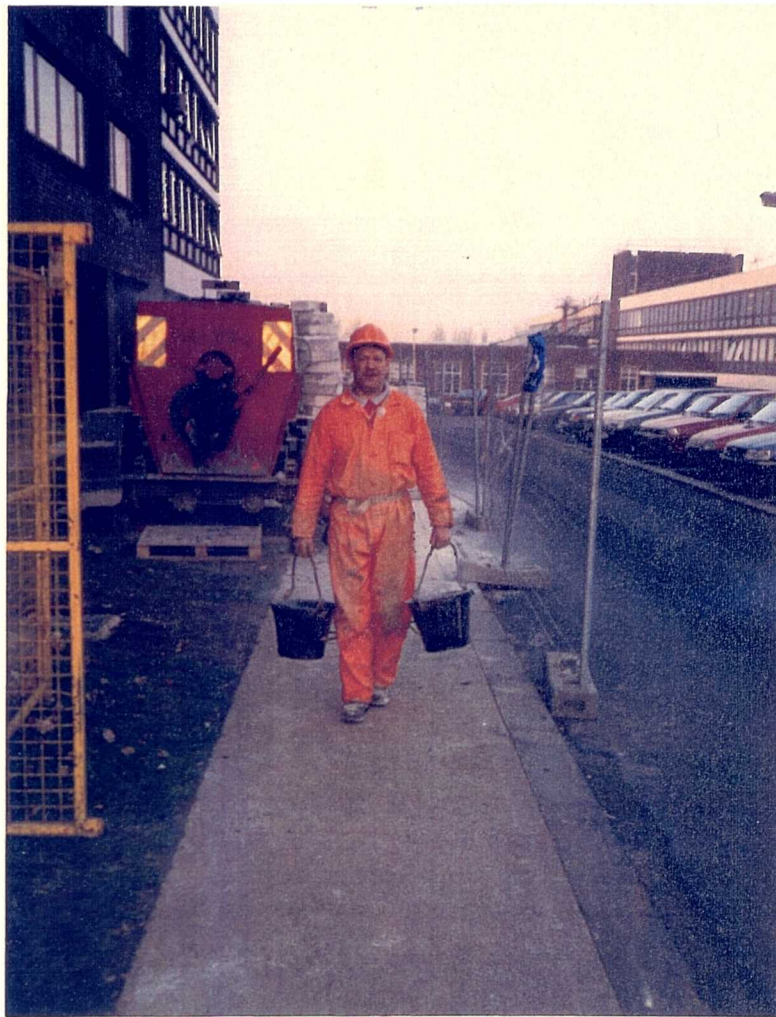
Figure : 11.2 c The Kettleman Has Emptied the Melted Mastic Asphalt in Buckets and Is Delivering Them Using the Lift Nearby
