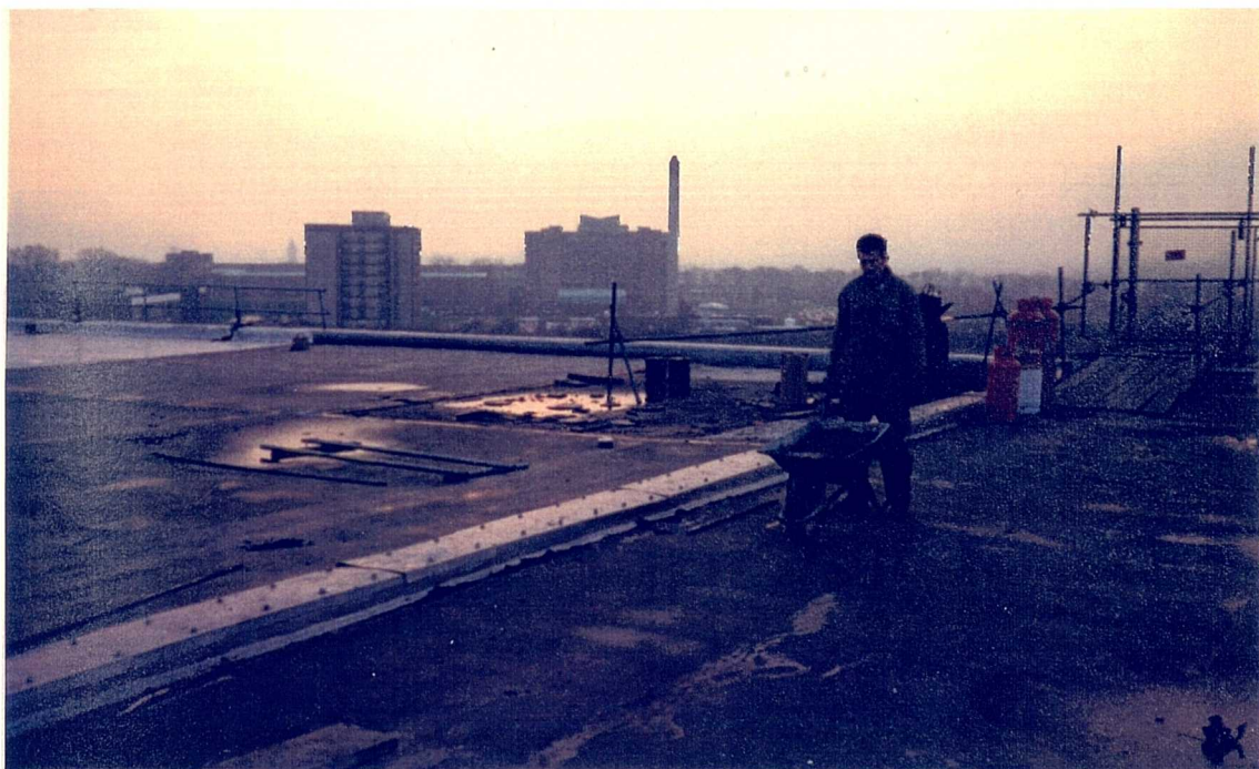
Figure : 11.2 d The Tipper is Delivering the Melted Mastic Asphalt to the Troweller Using the Wheelbarrow
