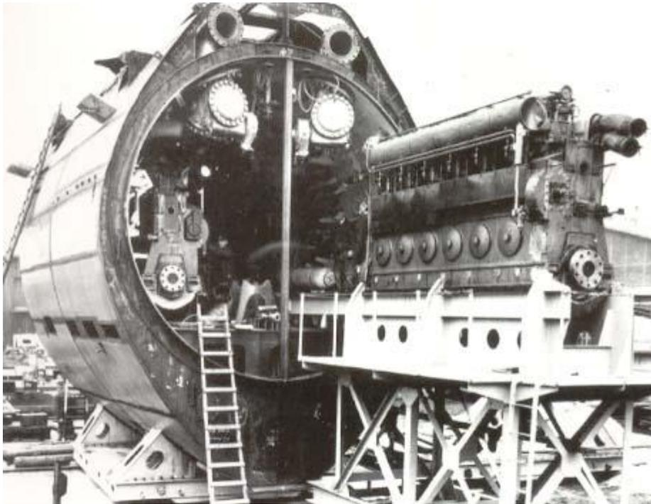
**Figure 2.2 - U-Boat construction in WWII, showing advanced blocks being used (source: forum.axisindustry.com)**
