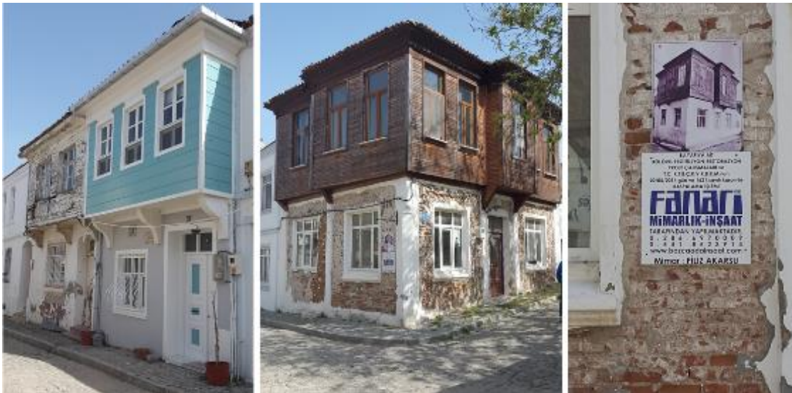
Figure 20: Examples of houses undergoing restoration (Okumus, 2015)
