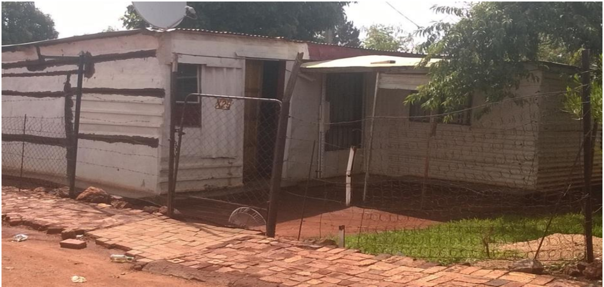
Figure 6.3: Shack house in the informal settlement
