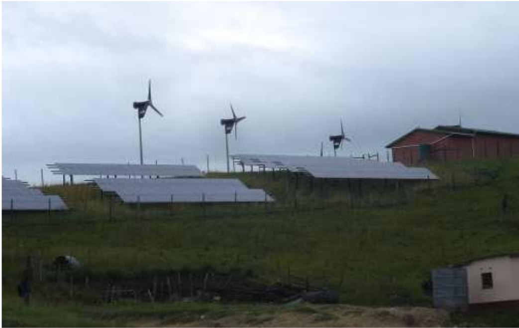
Figure E.2: The PV panels and wind generators in Lucingweni
