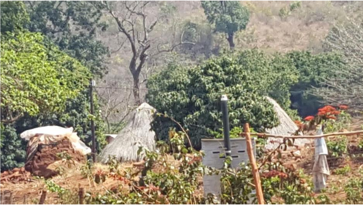
Figure 6.6: Electrified traditional thatched roof house in Elim village, Limpopo Province
