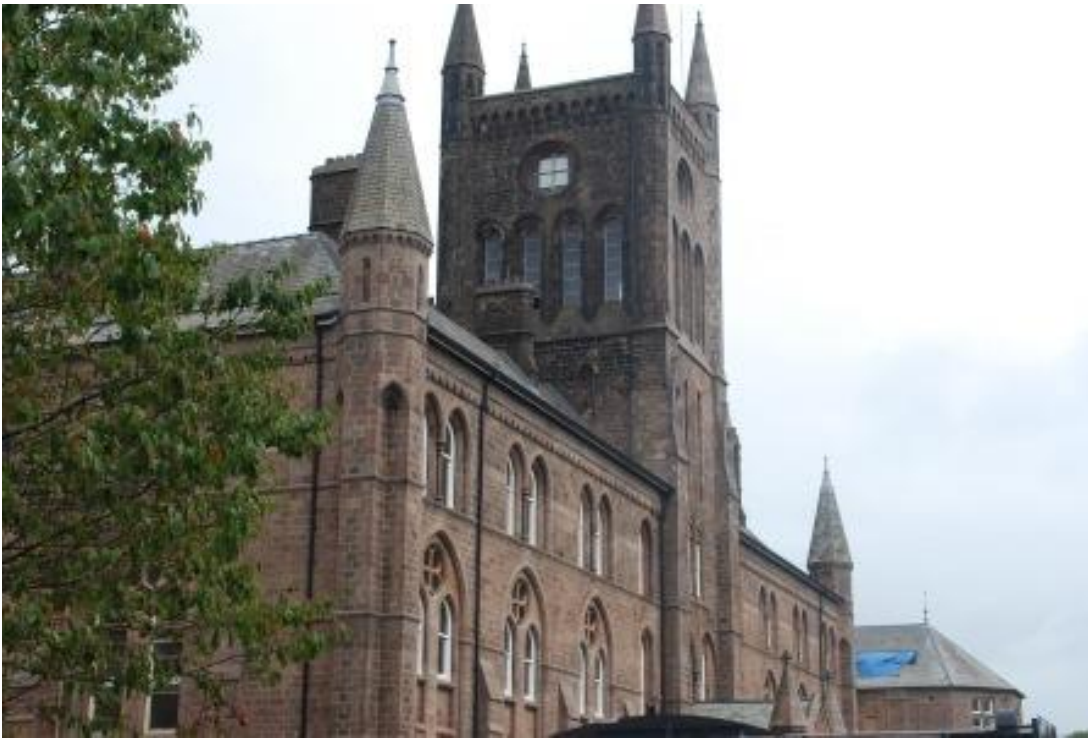
Figure 1.5: The main entrance of the Annexe, Lancaster Moor (author, 2014)
