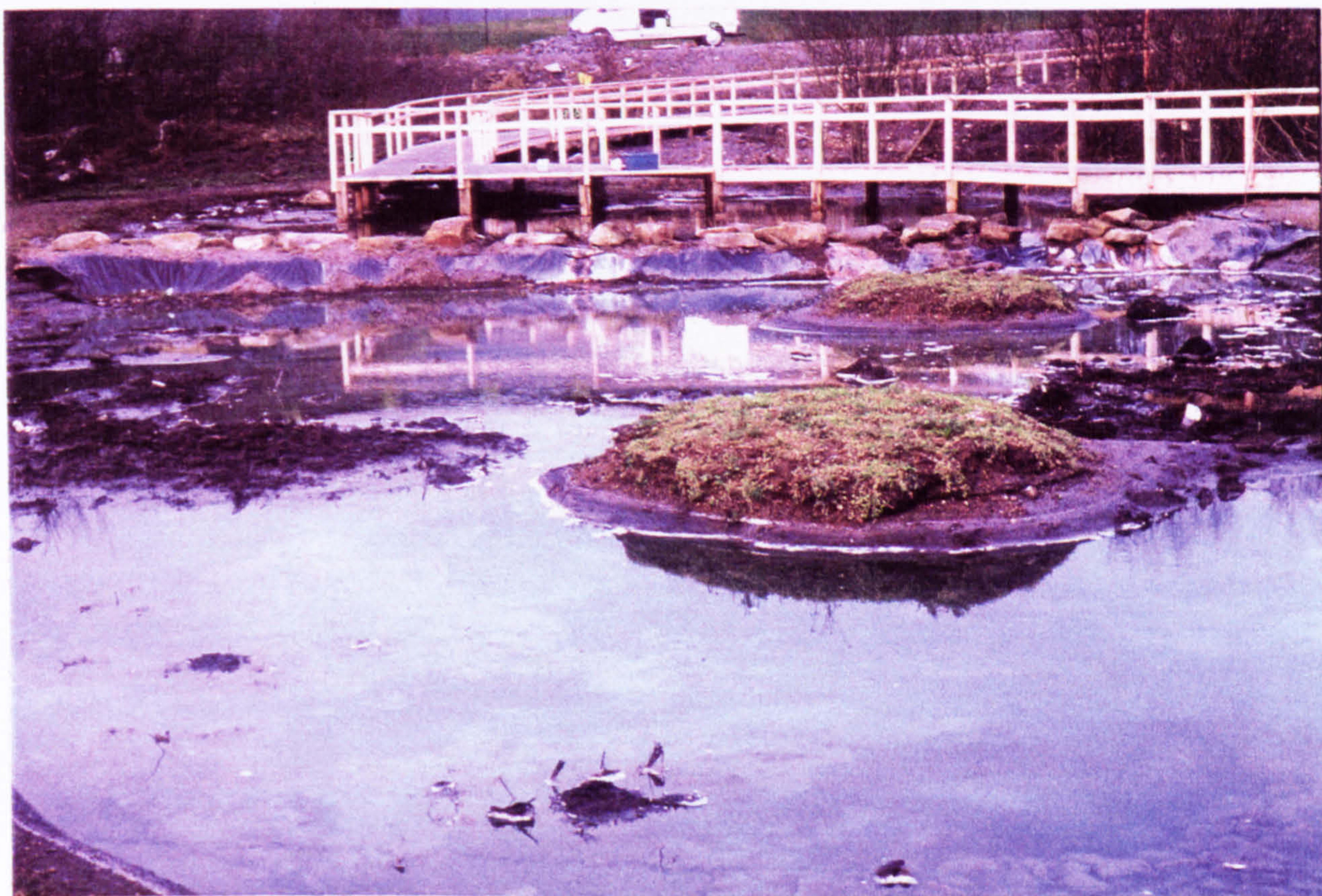
Figure 4.6 The footbridge and central weir of the Quaking Houses Community wetland (just in front of the footbridge) during its early operation (photograph by the author).
