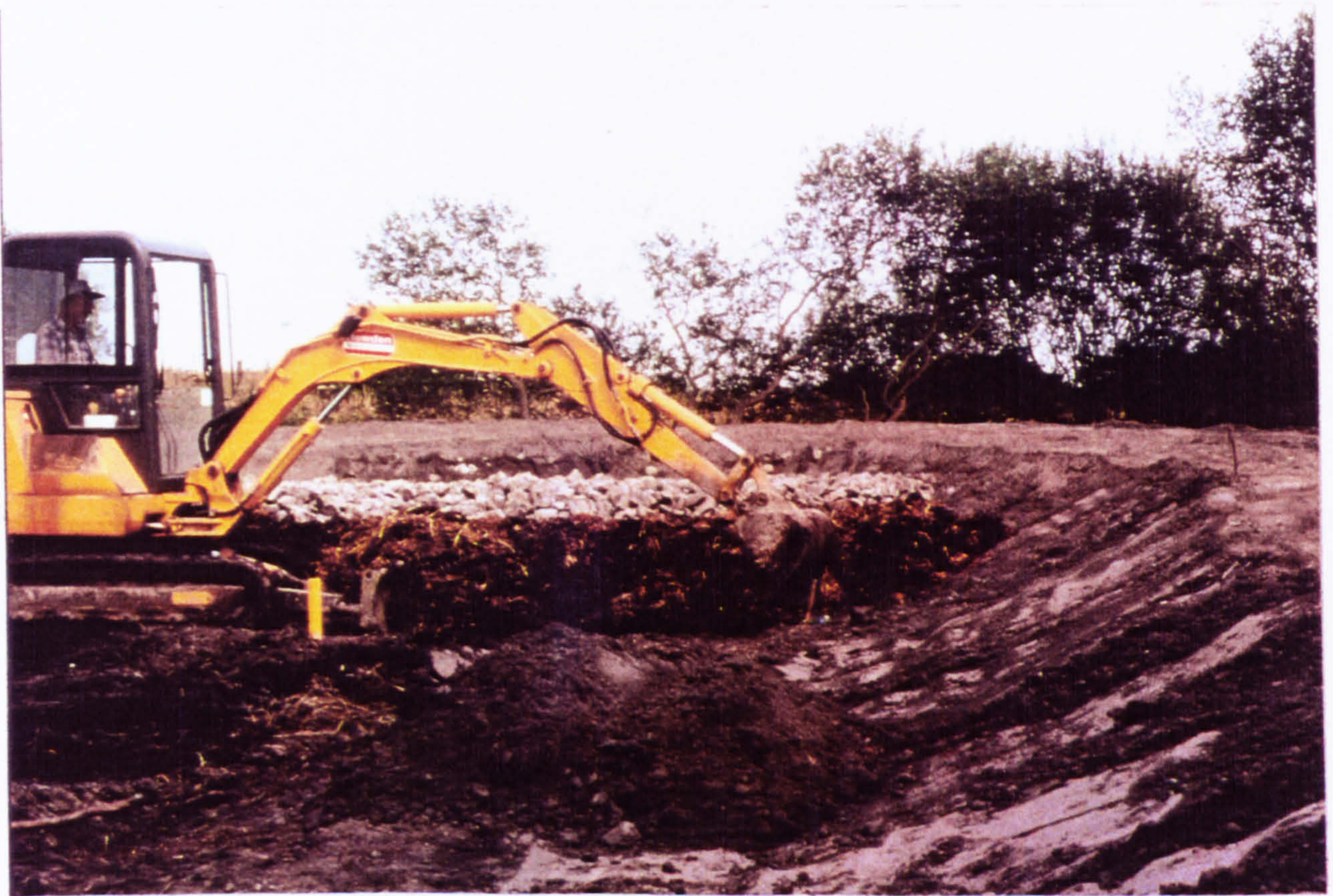
Figure 4.3 The pulverised fuel ash retaining embankment at Quaking Houses wetland under construction in the Summer of 1997 (photograph by the author).
