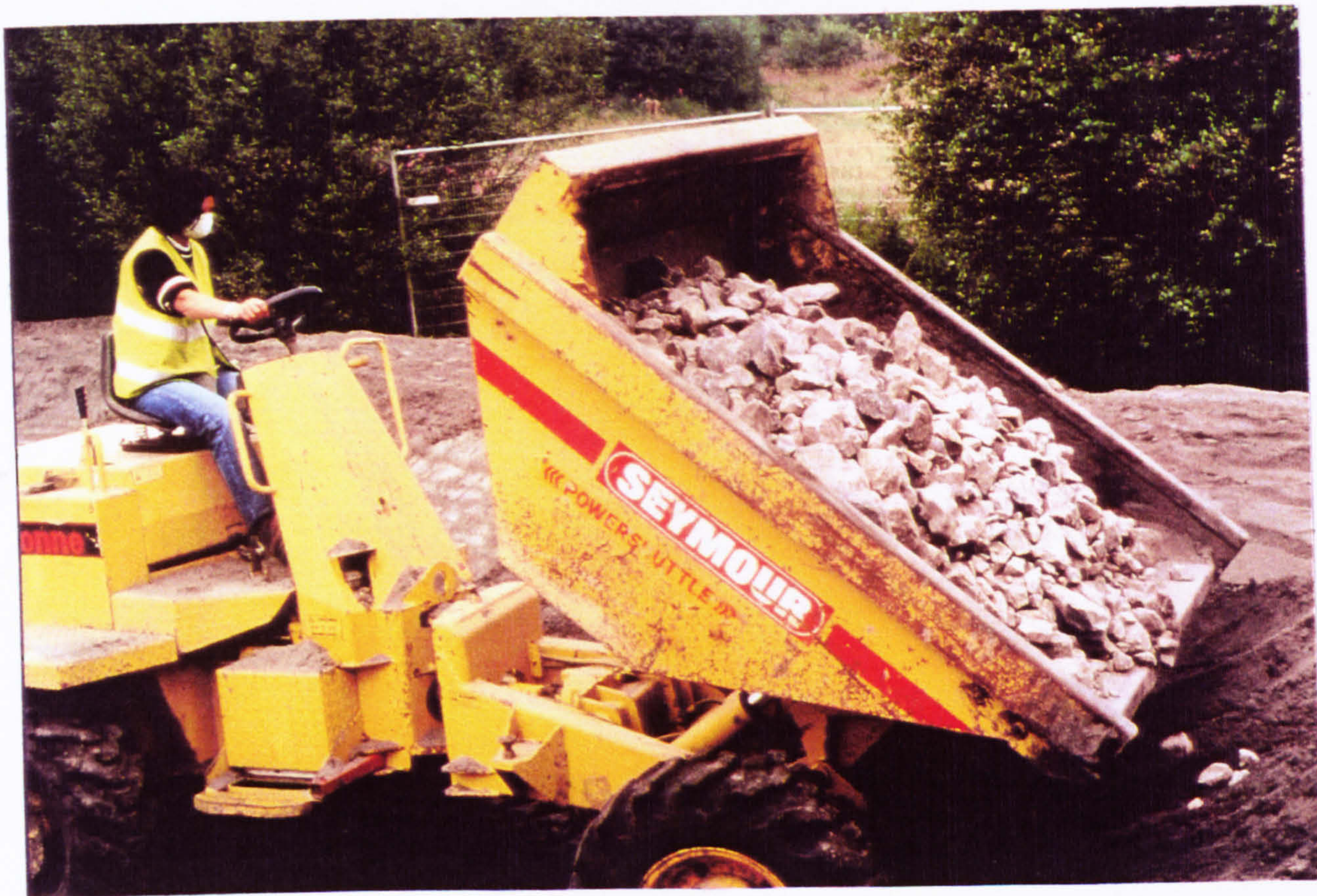
Figure 4.5 Limestone, for final pH adjustment, being placed at the far end of the Quaking Houses wetland in the Summer of 1997 (photograph by the author).
