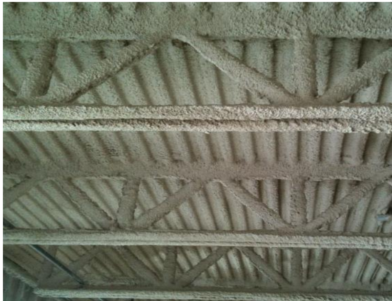
Figure 2.6 Example of fireproofing material sprayed onto steel structure ( http://southerninsulationgroup.com/sprayed-fire-resistive-material/ )
