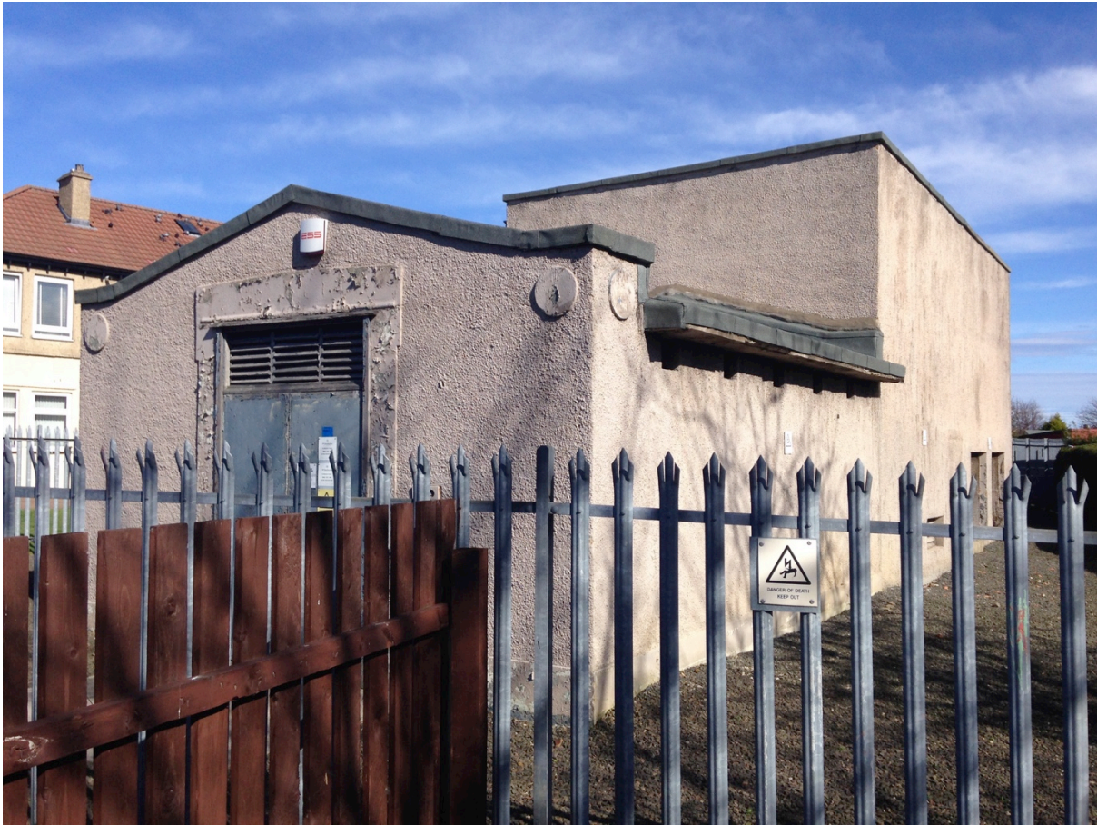
(Figure 5.11: Electricity substation located adjacent to LSG)
