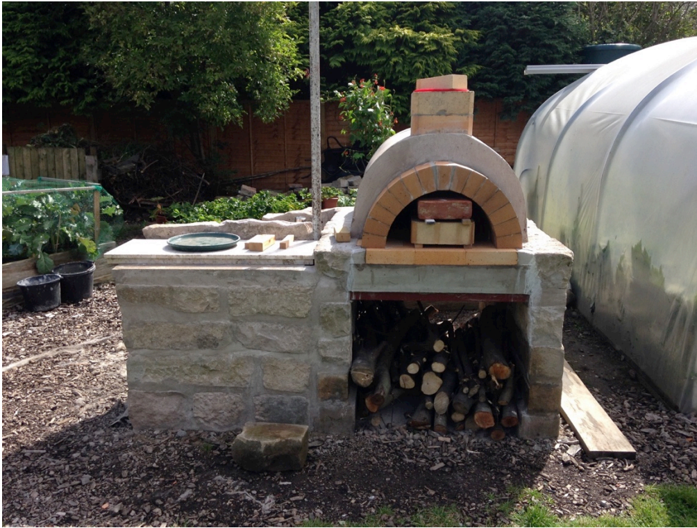
(Figure 7.7: Outdoor oven under construction at LSG)
