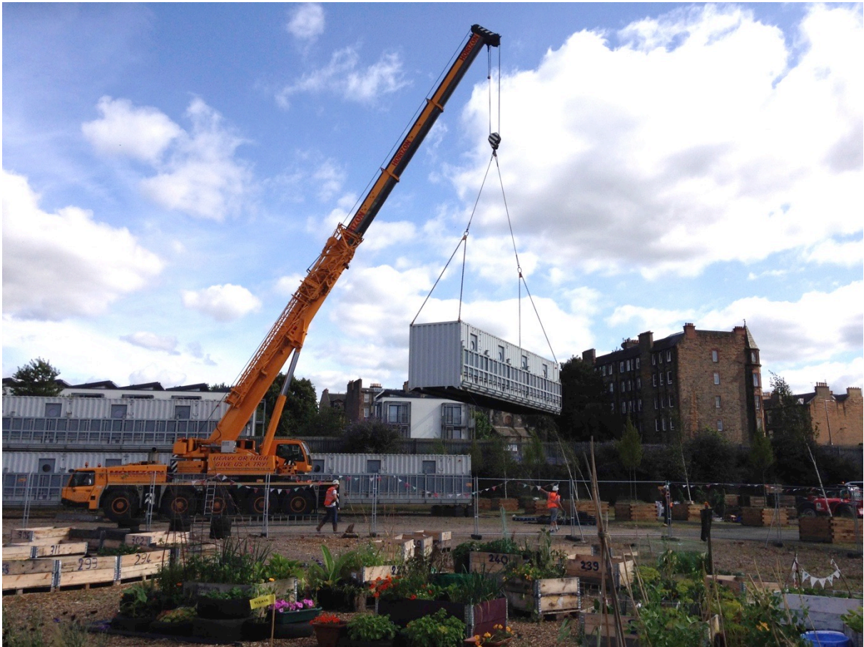
(Figure 5.10: Assembling the Snoozebox Portable Hotel, 21/07/14)
