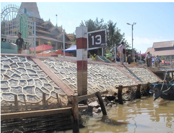
Picture 7.29: The banks of the Nyaungshwe to Inlay Lake channel have been concreted over, reducing habitat and increasing sediment flow, which affects the lake ecosystem.
