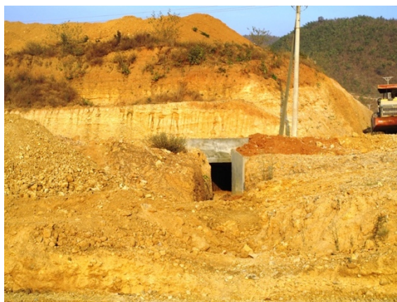
Picture 7.22: Construction of a road and box-culvert in the hotel zone.
