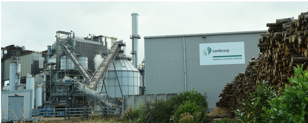
Figure 6.4 Photo of Wilton 10 power station
