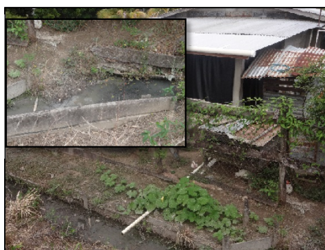
(b) A household disposing grey water on to an external drain within one of the sample communities.
