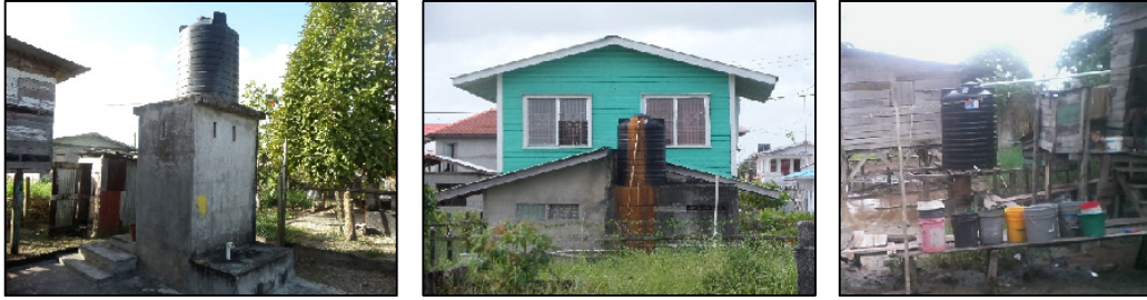
Figure 6-16. Variations of alternative water storage arrangements used by households in Guyana.
