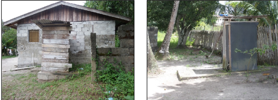
Figure 6-18. Pit Latrine with concrete chamber base in the town of Linden (Region 10)
