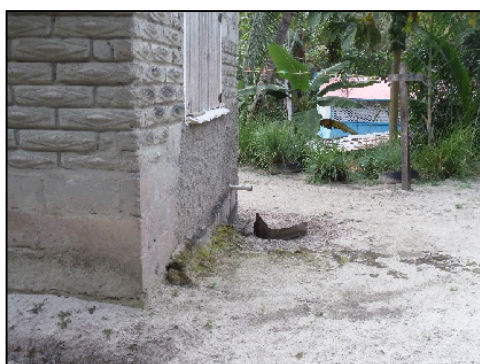
(a) A household disposing grey water onto the ground surface within their yard.
