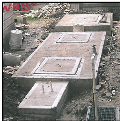
b) Concrete septic tank construction at a property in Barbados
