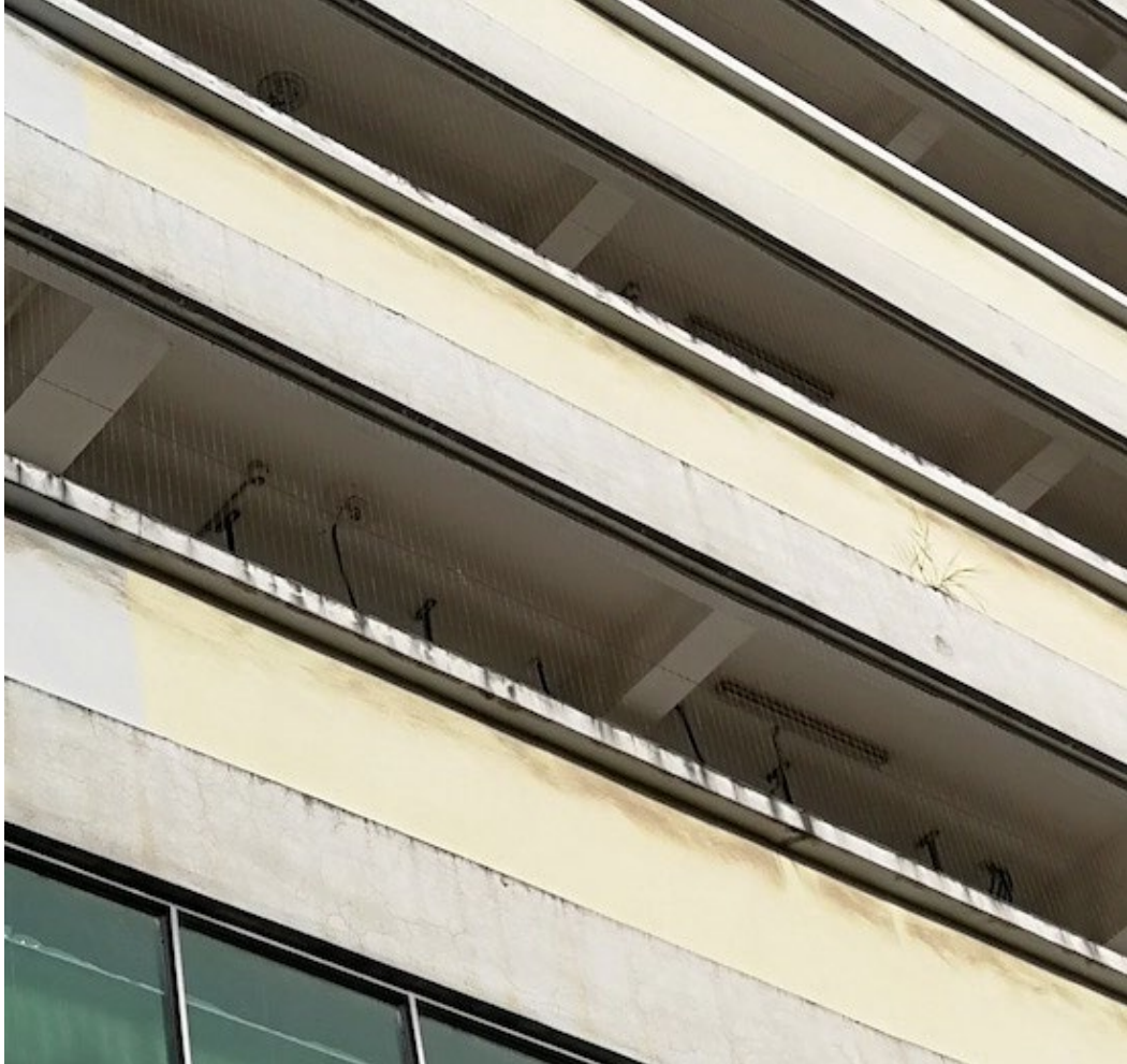
Figure 5-1. Mental nets installed in the Foxconn dormitories to prevent suicide Source: pictured by the author
