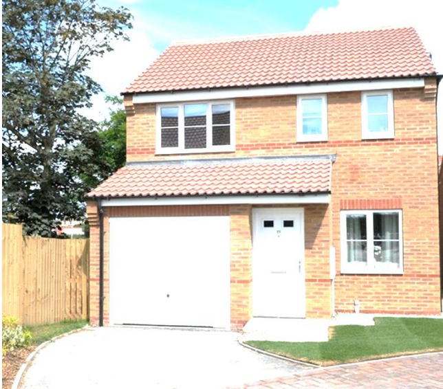
Figure 60: Domestic residential case for Newcastle
