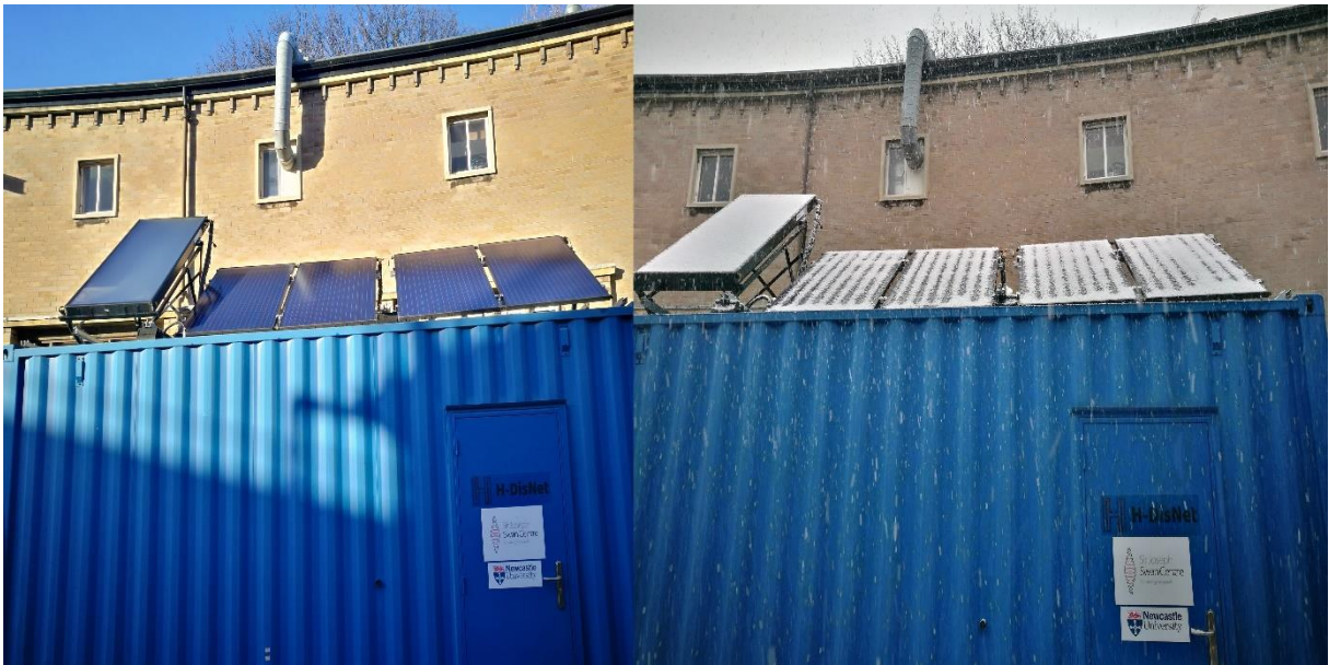
Figure 55: Lab unit setup in snow and sunny conditions
