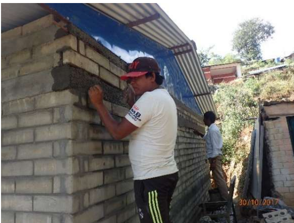
Figure 4-29 - Local labourers constructing a CSEB house in rural Sindhupalchowk. CSEB was also used to construct the village school, sharing the skills learnt.
