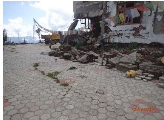
Figure 4-13 - Soft-storey failure of a temple in rural Sindhupalchowk.
