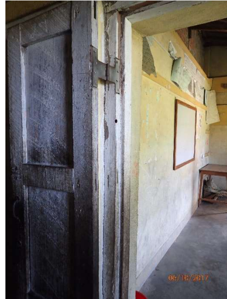
Figure 4-11 - Flush hinges on a classroom door at first SESP retrofitted school. These create less obstruction in the doorway, making it easier to evacuate.
