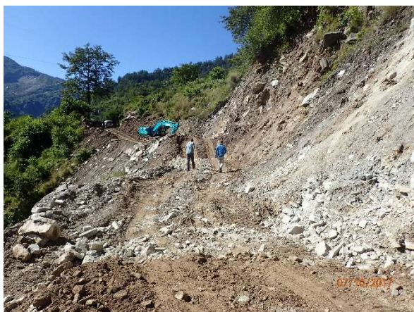
Figure 5-5 - A seasonal road being reconstructed following a landslide, using an excavator (seen back left of the image).
