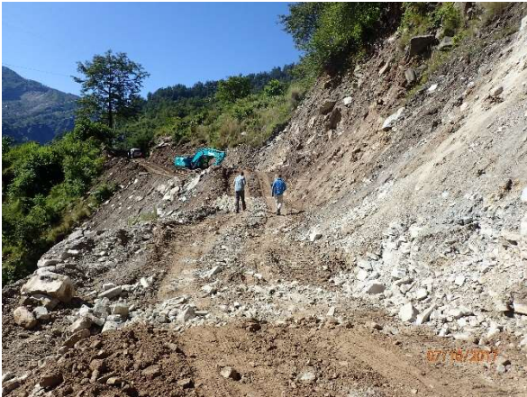
Figure 10 - A seasonal road being reconstructed following a landslide, using an excavator (seen back left of the image).
