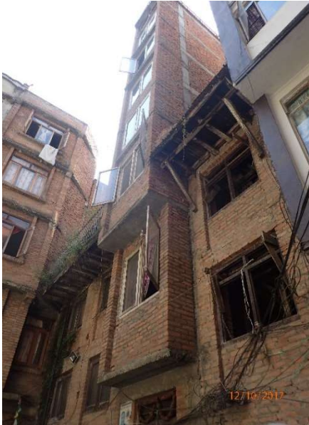
Figure 4-10 - Residential buildings in Patan, extended vertically, often without suitable engineering input, and is likely to cause structural inadequacies.
