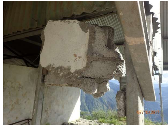
Figure 4-21 - Earthquake damage to a school in rural Sindhupalchowk. There was out of plane failure of the wall panels, due to poor connection to the steel frame.
