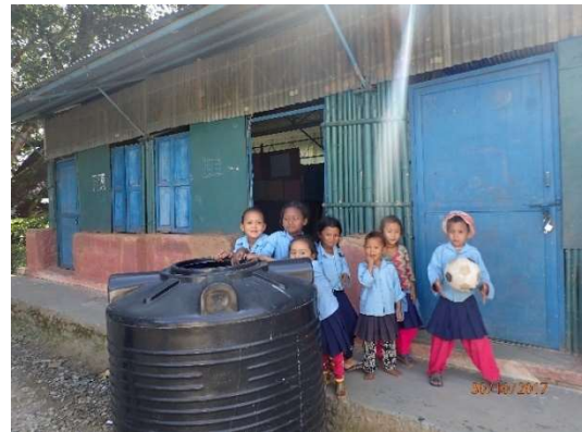
Figure 2-4 - Temporary Learning Centre, at a school visited during the pilot study field visit, constructed on the original foundations using bamboo and CGI sheeting for the roof.
