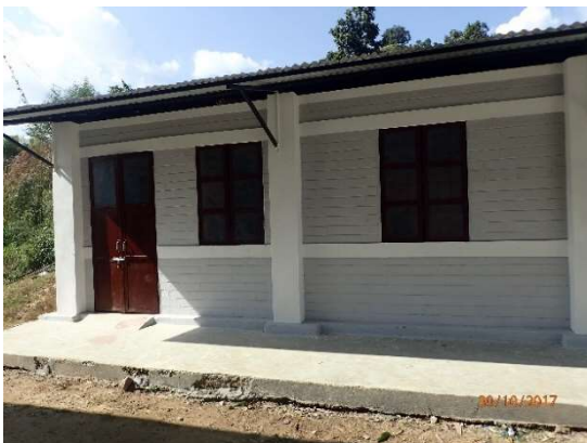
Figure 4-26 - RC frame with CSEB infill wall, in rural Sindhupalchowk.
