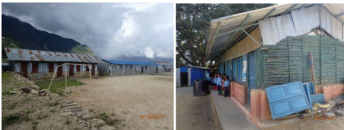
Figure 4-22 - A Temporary Learning Centre, providing additional learning spaces at a damaged school in rural Sindhupalchowk, constructed with CGI sheeting. Figure 4-23 - A Temporary Learning Centre at a case-specific school in rural Sindhupalchowk, constructed with bamboo and CGI sheeting.
