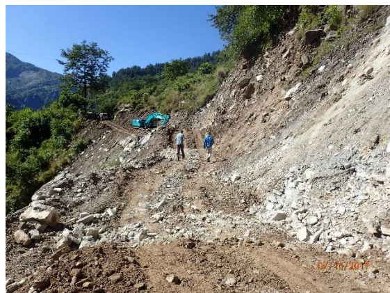
Figure 4-17 - A rural road under construction in rural Sindhupalchowk, using an excavator to cut the road out of the side of a slope face.
