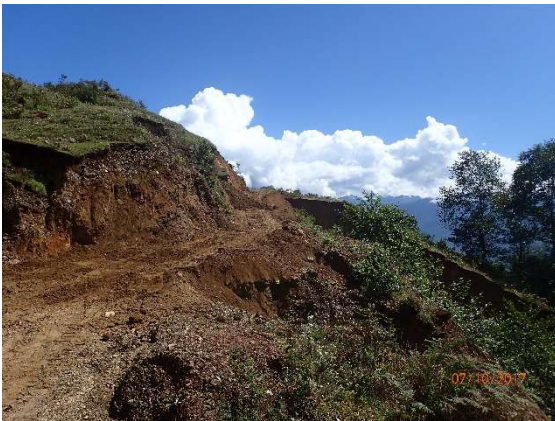
Figure 4-16 - A rural road in Sindhupalchowk, cut into a soil slope face - these roads are non-engineered and are often unstable.
