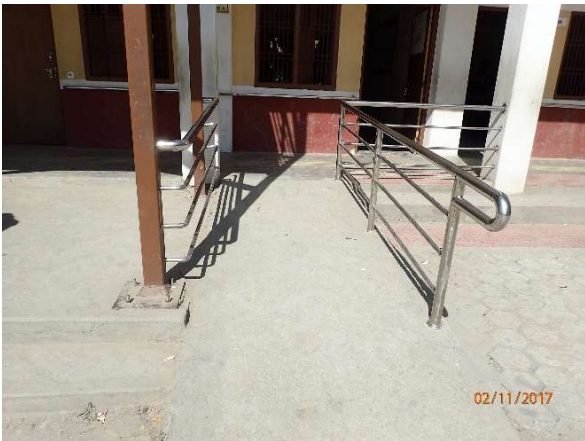
Figure 4-37 - An accessible ramp constructed at an urban school in the outskirts of Kathmandu.
