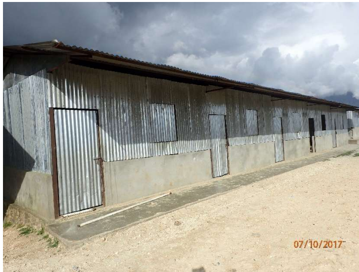
Figure 1 - A Temporary Learning Centre in Sindhupalchowk, constructed using timber and corrugated sheets, built on the existing foundations of the damaged school, visited during fieldwork conducted in Nepal.
