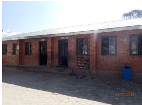
Figure 4-25 - A fired brick school building, constructed in the outskirts of Kathmandu.
