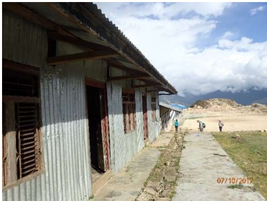
Figure 2-3 - Temporary Learning Centre, at a school visited during the pilot study field visit, constructed on the original foundation using CGI sheeting for both walls and roof.
