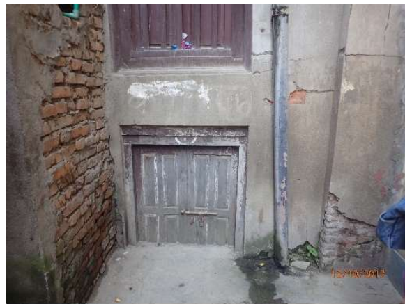
Figure 4-9 - Construction on top of debris from previous disasters, blocking exits from buildings.
