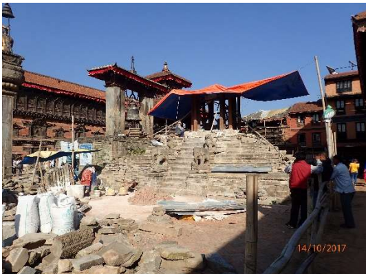
Figure 4-12 - Reconstruction of a temple in Bhaktapur, replicating traditional construction methods.
