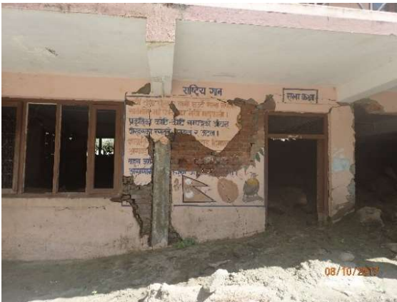
Figure 4-20 - A school in rural Sindhupalchowk, buried in mud, as the school sits in the path of a debris flow - a secondary effect of the 2015 Gorkha earthquake.
