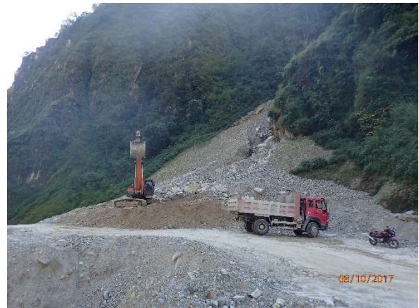
Figure 4-34 - Reconstructing a road that had buried in a landslide, blocking transport routes. Landslides caused by the monsoon can cut off many roads each year.
