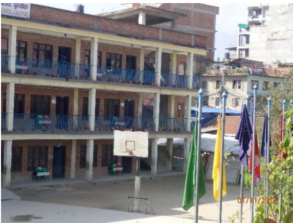
Figure 4-24 - RC frame and fired brick infill wall school, constructed in Kathmandu.
