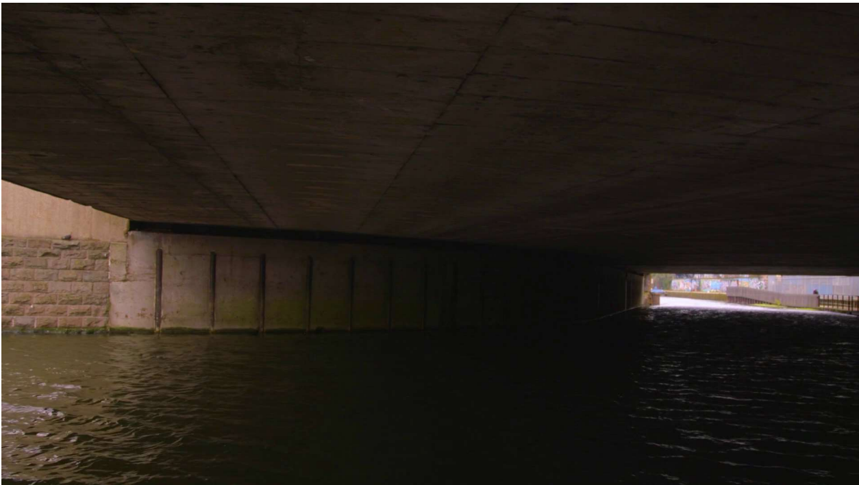
Figure 2. Beneath Bow Interchange in Lea River Bridges
