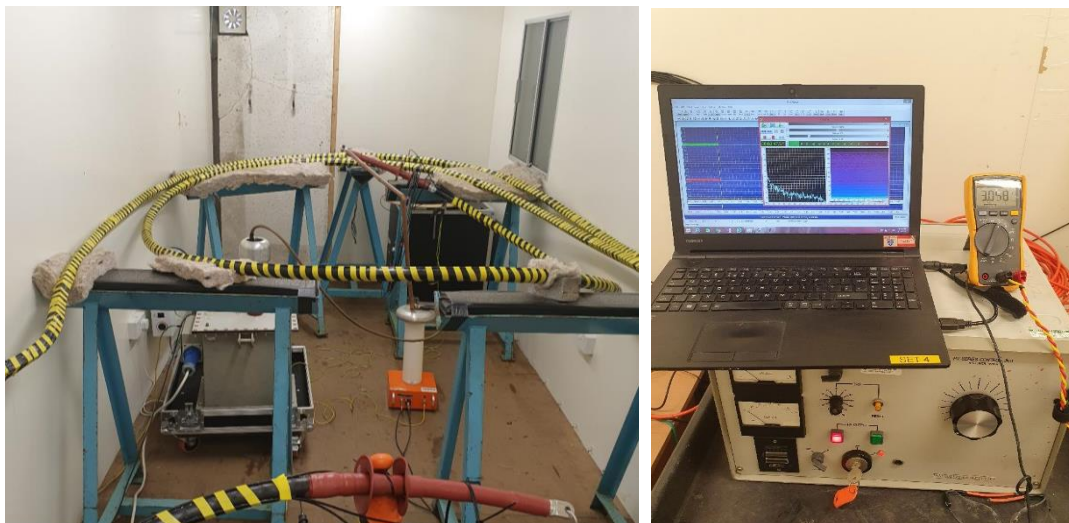
Figure 4- 24: Comparative Electrical PD Test Setup – Acoustic and Electrical Monitoring
