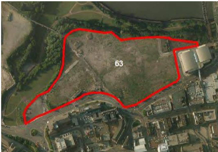
Figure 7-11 Location of former Vaux Brewery site, Sunderland
