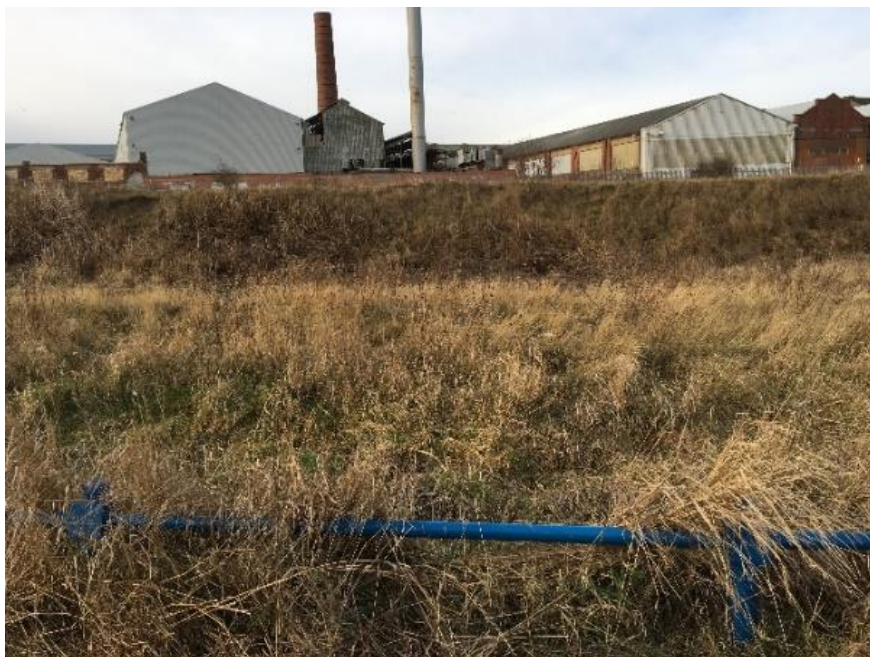
Figure 7-9 Former paper mill, Sunderland
