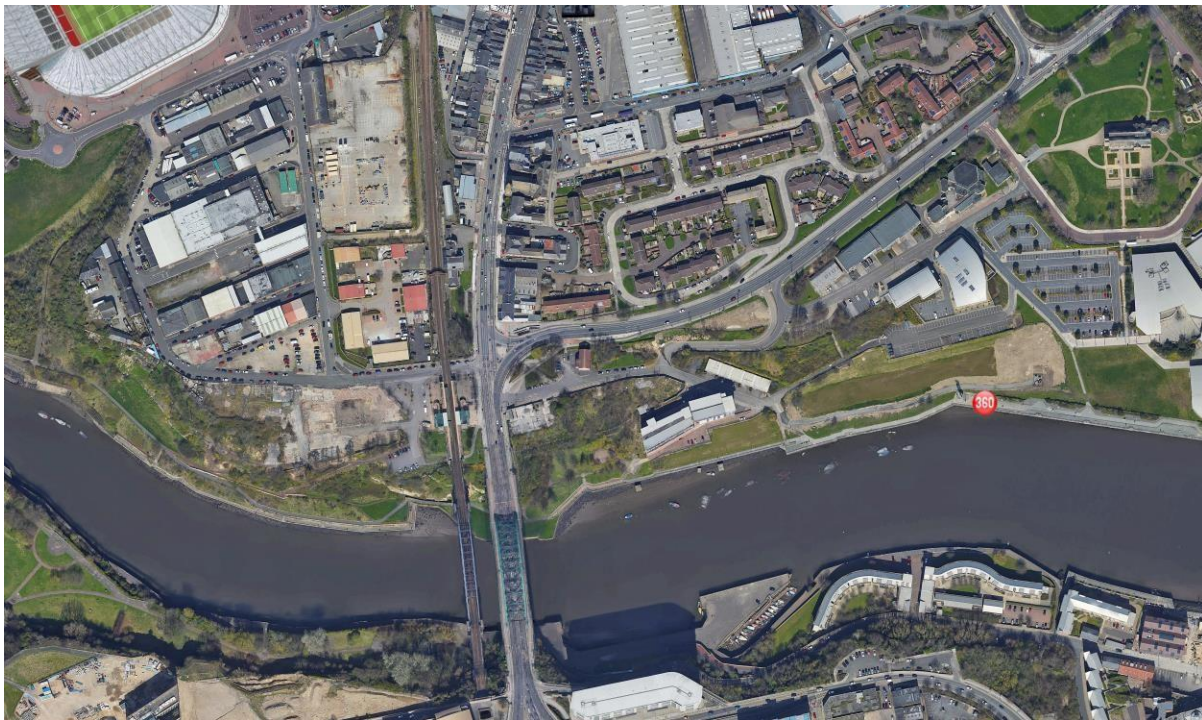
Figure 6-6 Former shipyard, Sunderland
