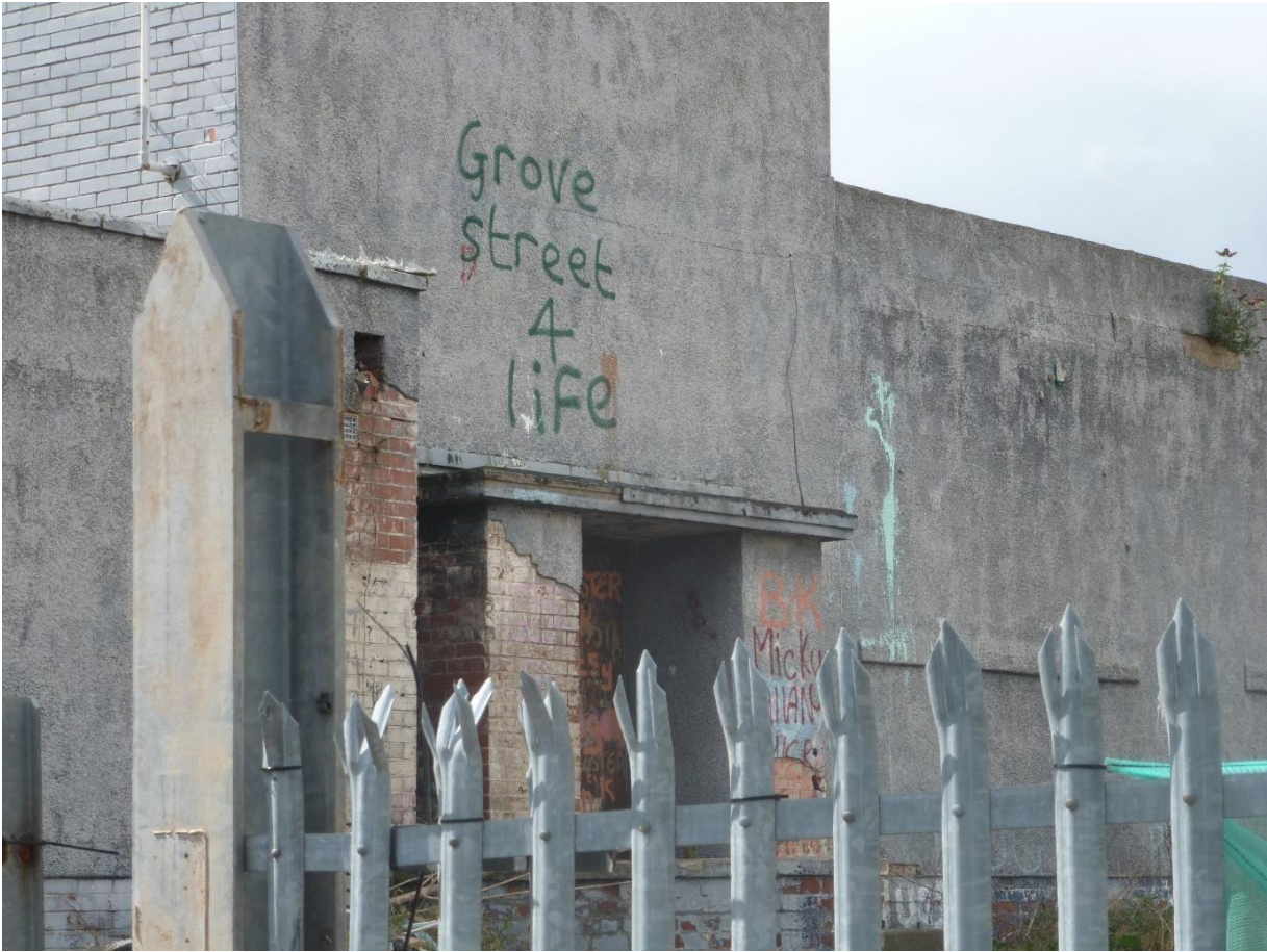
Figure 6-8 Former factory unit, Sunderland
