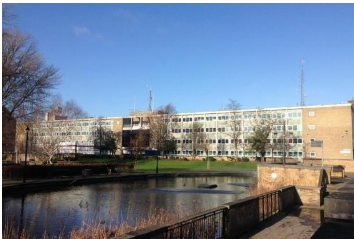
Figure 6-11 Former Police Station, Hull
