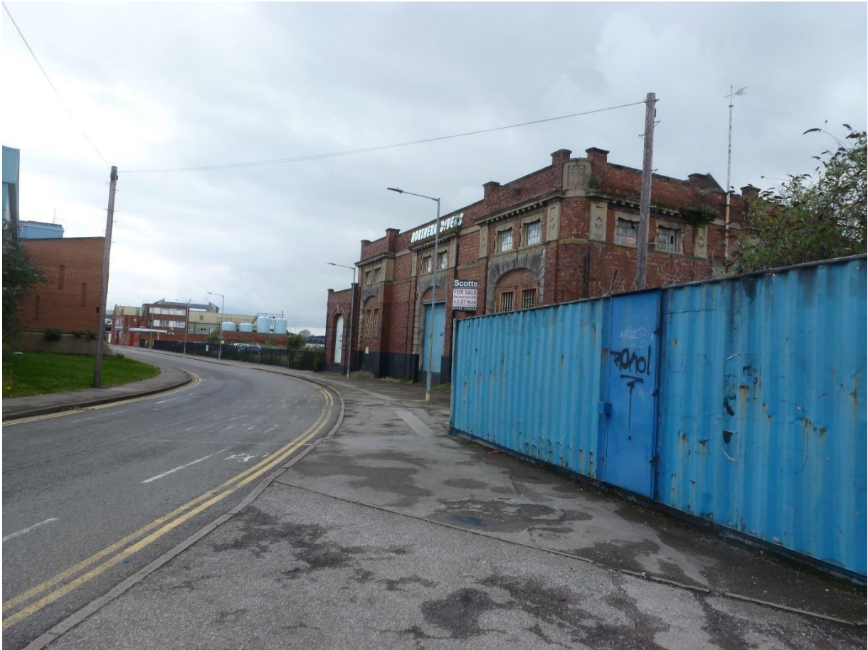
Figure 6-7 Former Northern Diver factory
