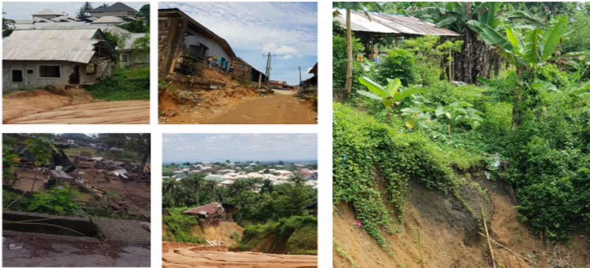
Figure 8.11: These photos show part of the access roads cut by erosion in Ikot Ansa
