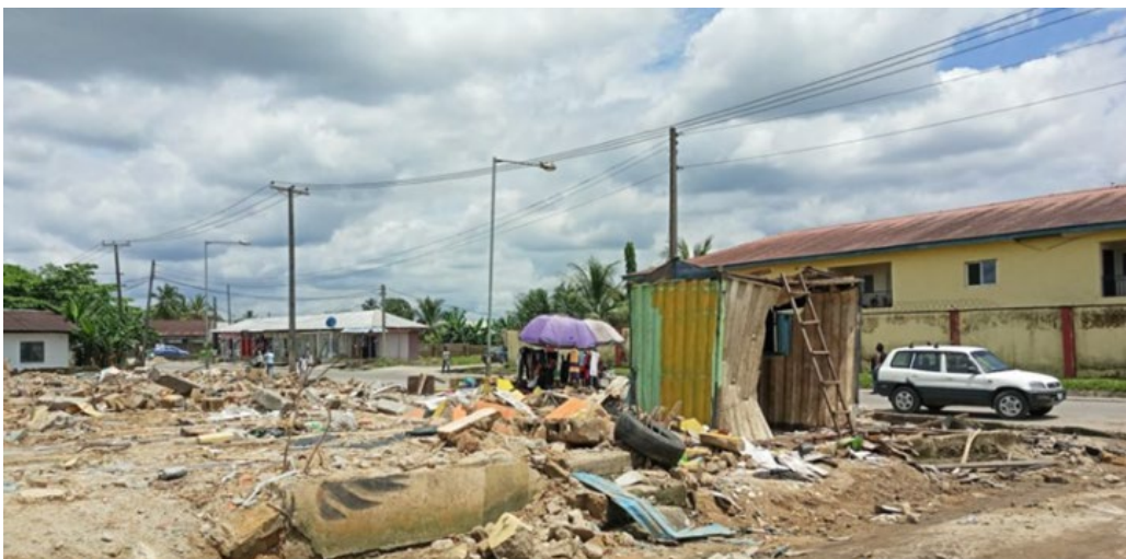
Figure 6.3: Demolition of squatter housing in Ikot Ansa.
