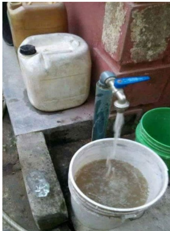
Figure 8.5: Water pump installed by the water board
