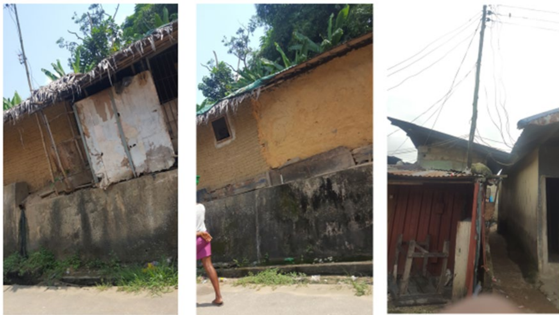
Figure 8.4: A typical house built with wood and mud in the study area
