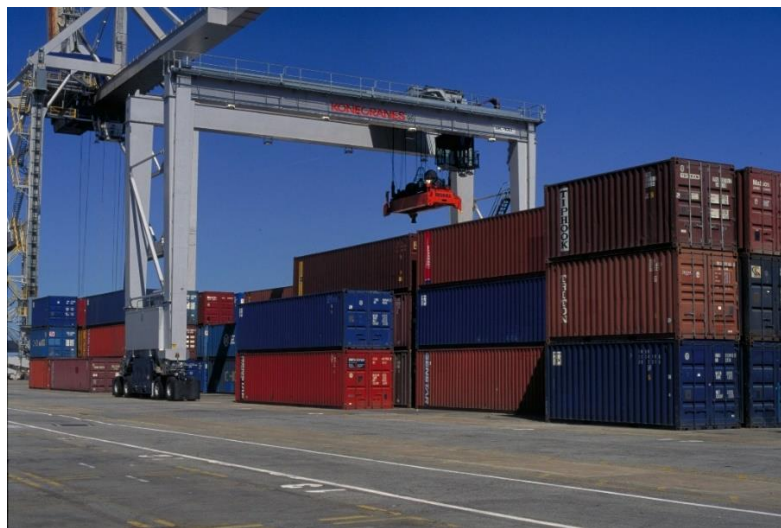
Figure 2.9: Automated Rubber Tired Gantry (ARTG) System
