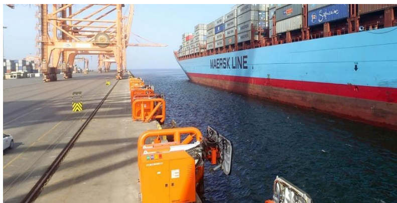
Figure 2.8: Automated Mooring System (AMS)
