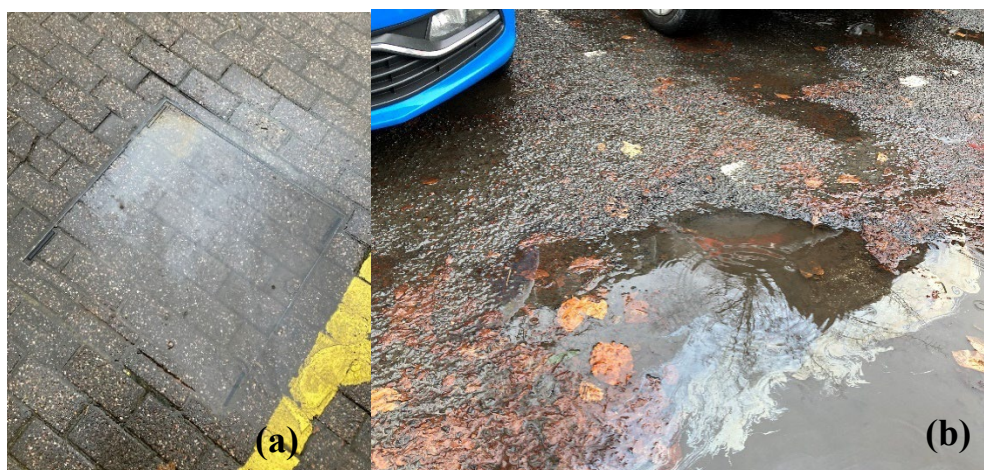
Figure 2.4. Oil pollution on the permeable (a) and impermeable (b) pavement of car parks after rain.
