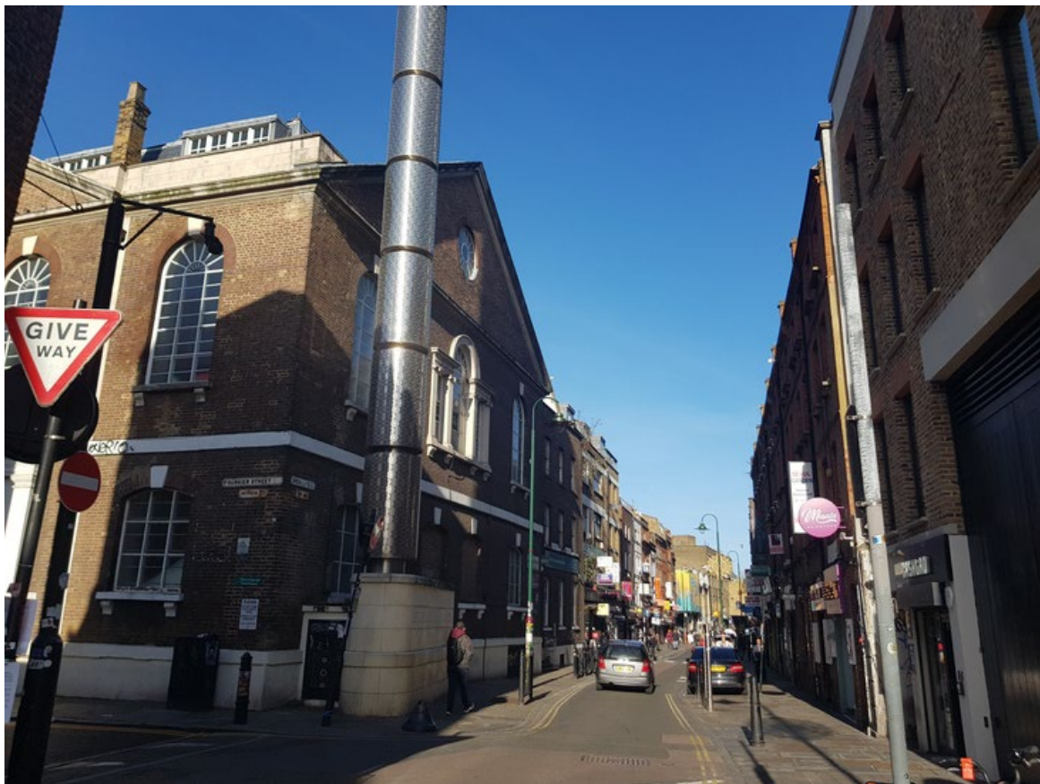
Figure 14: The Brick Lane Mosque
