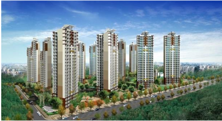
Figure 3-4 Bird's-eye view of Bangbae Arhill (Raemian construction, 2004)
