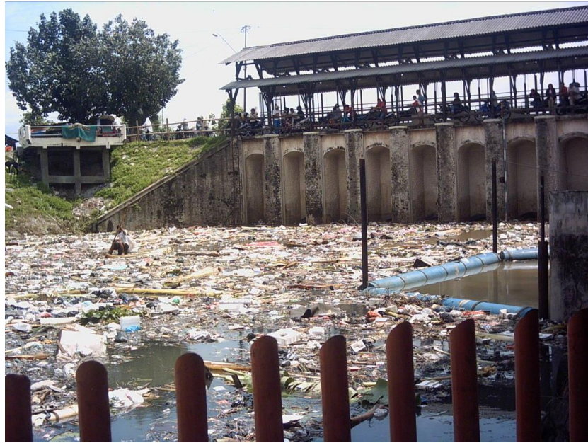
Figure 3. 12. Solid waste blocking the weir in the upper reach of Bengawan Solo River (source : Surakarta Public Work Agency)
