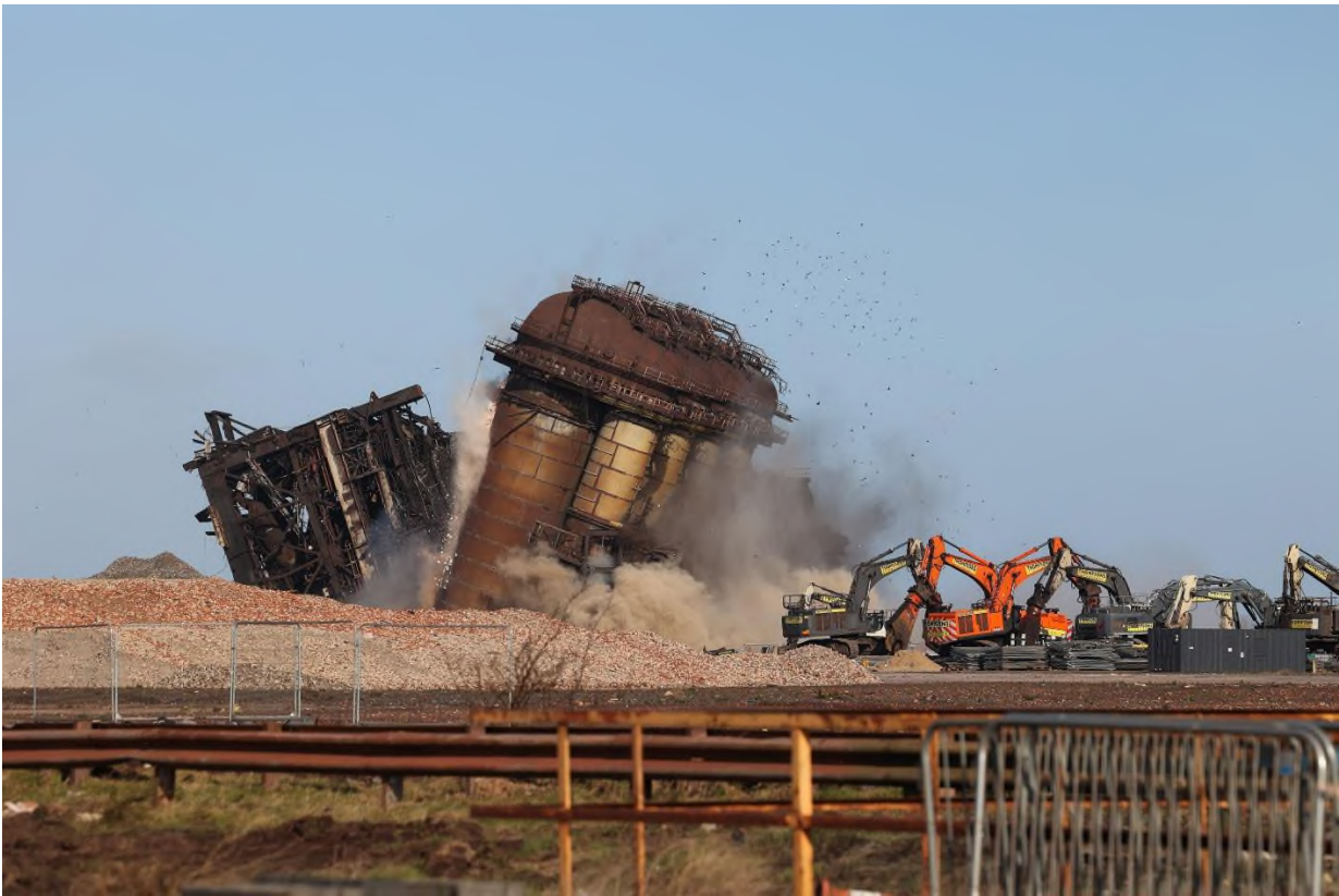
Figure 41: Demolition of Redcar Blast Furnace
