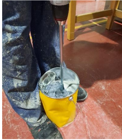
(h) These two components are mixed in a ratio of 3:1 until a uniform light grey colour is achieved.
