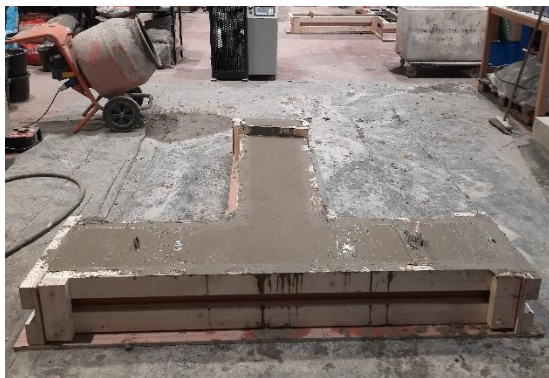
(k) Pouring concrete
