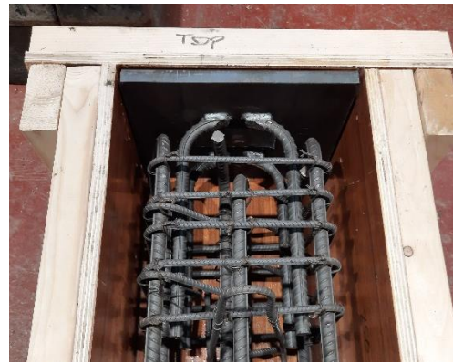
(j) Column upper end detail (sketch of the support details were given in Chapter 3.6)
