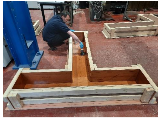
(b) Vanishing of formworks
