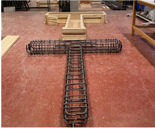
(g) Combining column and beam reinforcements
