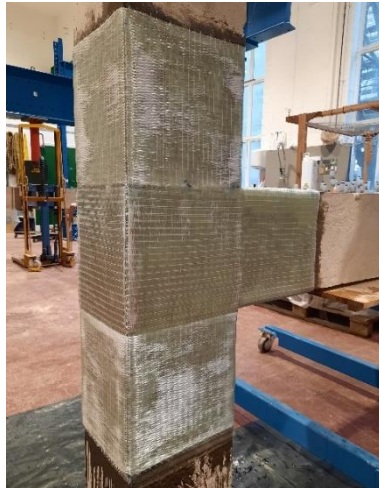
(g) Application completed column-beam joint
