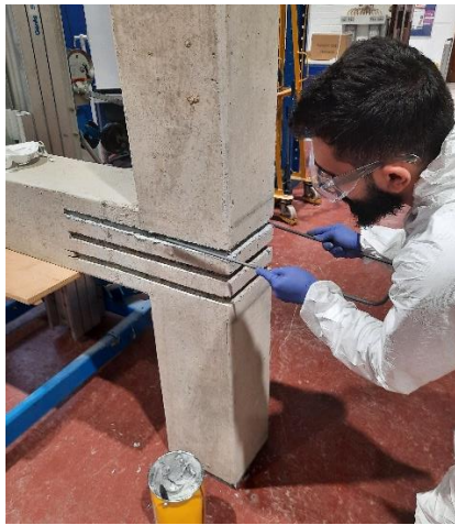
(i) Filling the grooves halfway with epoxy and then inserting the steel bar into the groove and pressing it gently.
