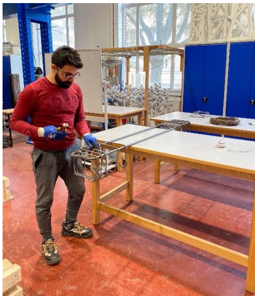
(e) Tying of the column reinforcements
